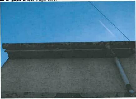
Soffits are well sealed and close fitting with no gaps.
