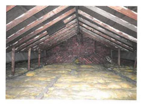
Underfelt is all in good condition with no rips or tears. No gaps or crevices are present in interior brickwork within the loftspace.
