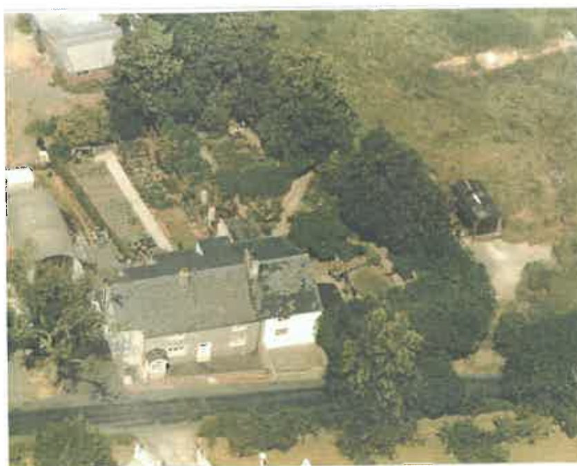
Photograph 2 – Ariel photograph of the existing building and building behind
