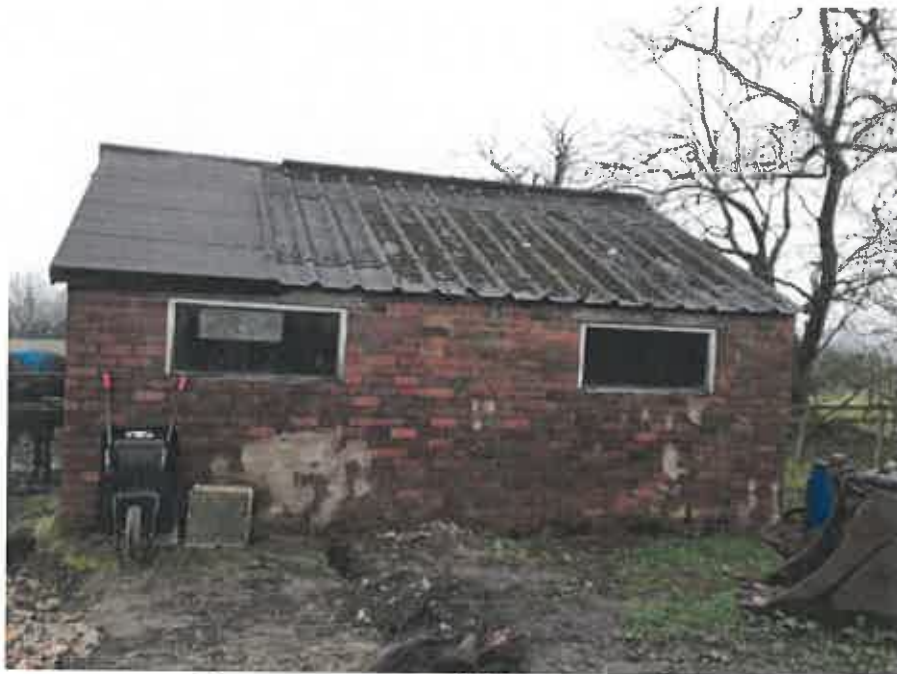
Photograph 1 – Building to be converted
