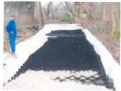
Installation of the CellWeb™ system.
