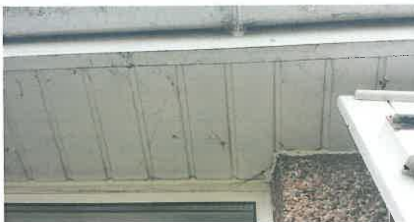
Tight fitting nature of soffits
