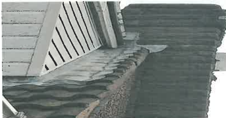
Mortar filled ridge
