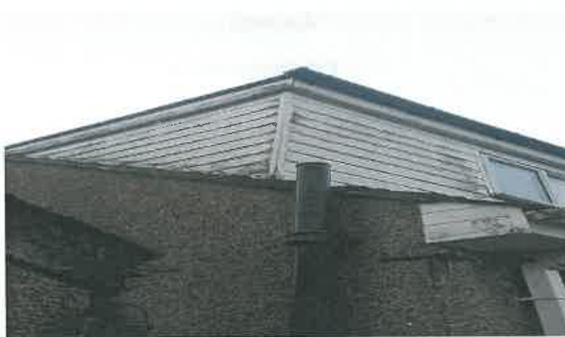
PVC cladding on dormer
