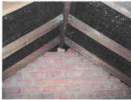
Figure 5: main roof void
