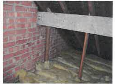
Figure 6: main roof void
