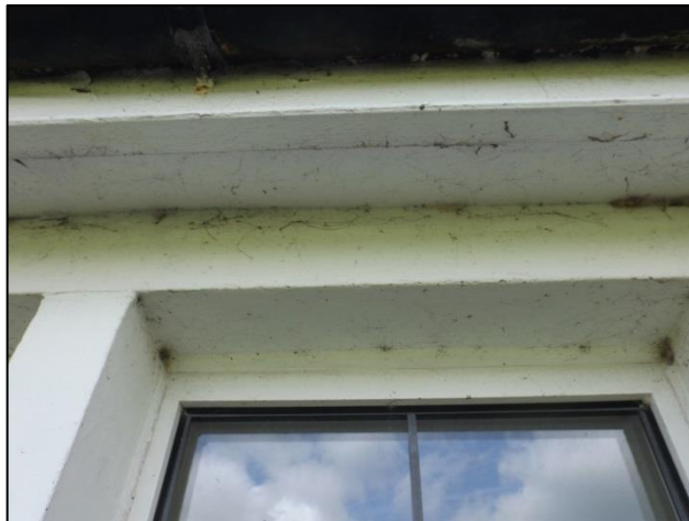
Plate 5: The eaves were completely sealed up with no potential for bat access.
