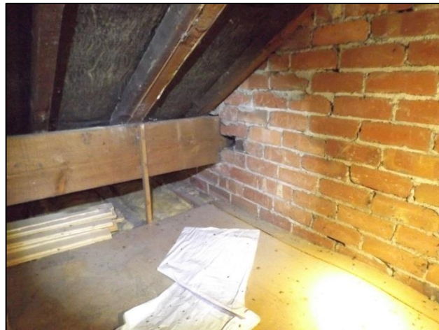
Plate 18: Gaps in the brickwork were large enough for bats to acquire access to the loft void.
