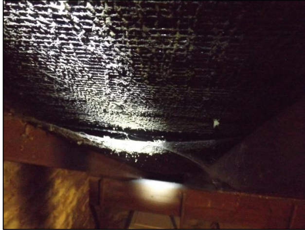
Plate 17: There were voids behind the bitumen felt that may provide resting places/access to bats.
