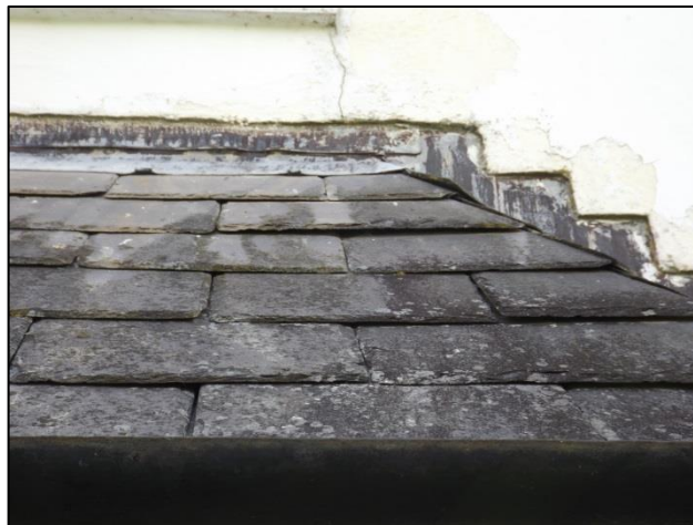
Plate 11: The bay window at the rear also had gaps in the slate tiles.
