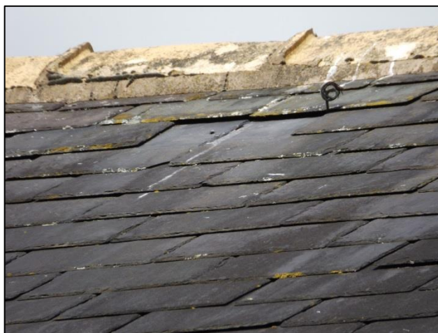
Plate 9: Missing tiles on the eastern aspect of the pitched roof.
