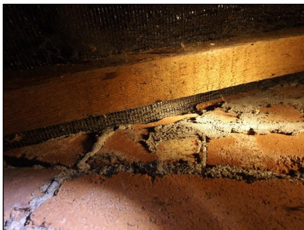
Plate 19: There were spaces between the brickwork and the felt large enough to allow access.
