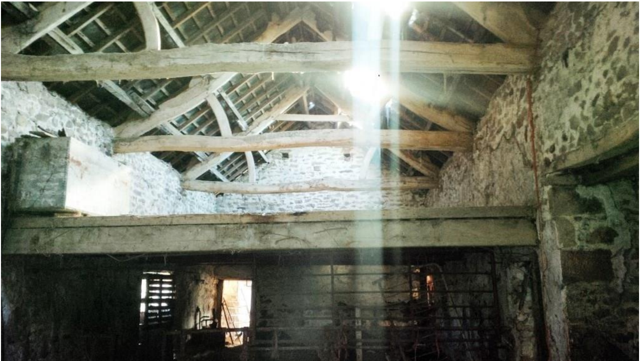
Figure 10. Interior of original barn looking south showing inserted loft floor and original trusses with trenced purlins, struts and upper ties
