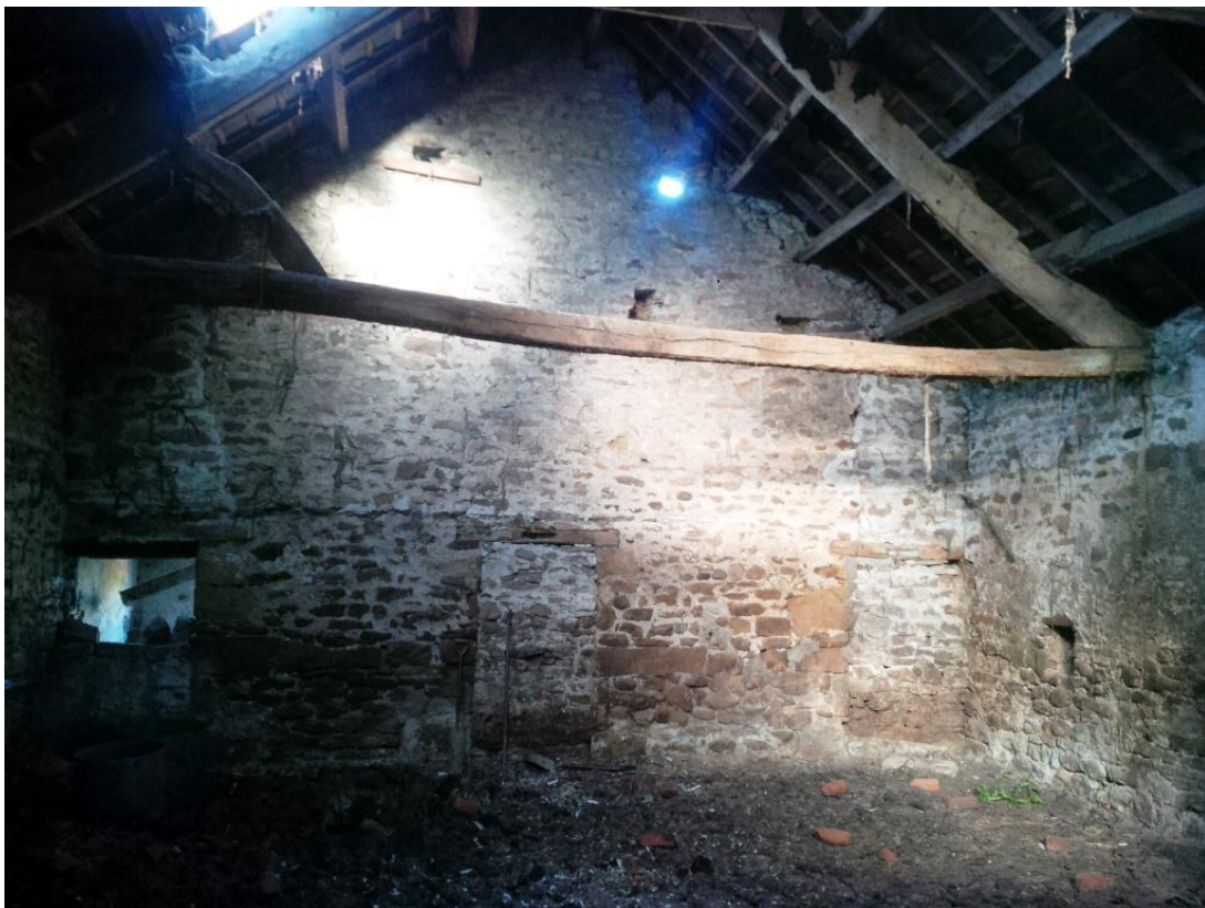
Figure 9. Interior of original barn showing blocked former northern gable doors
