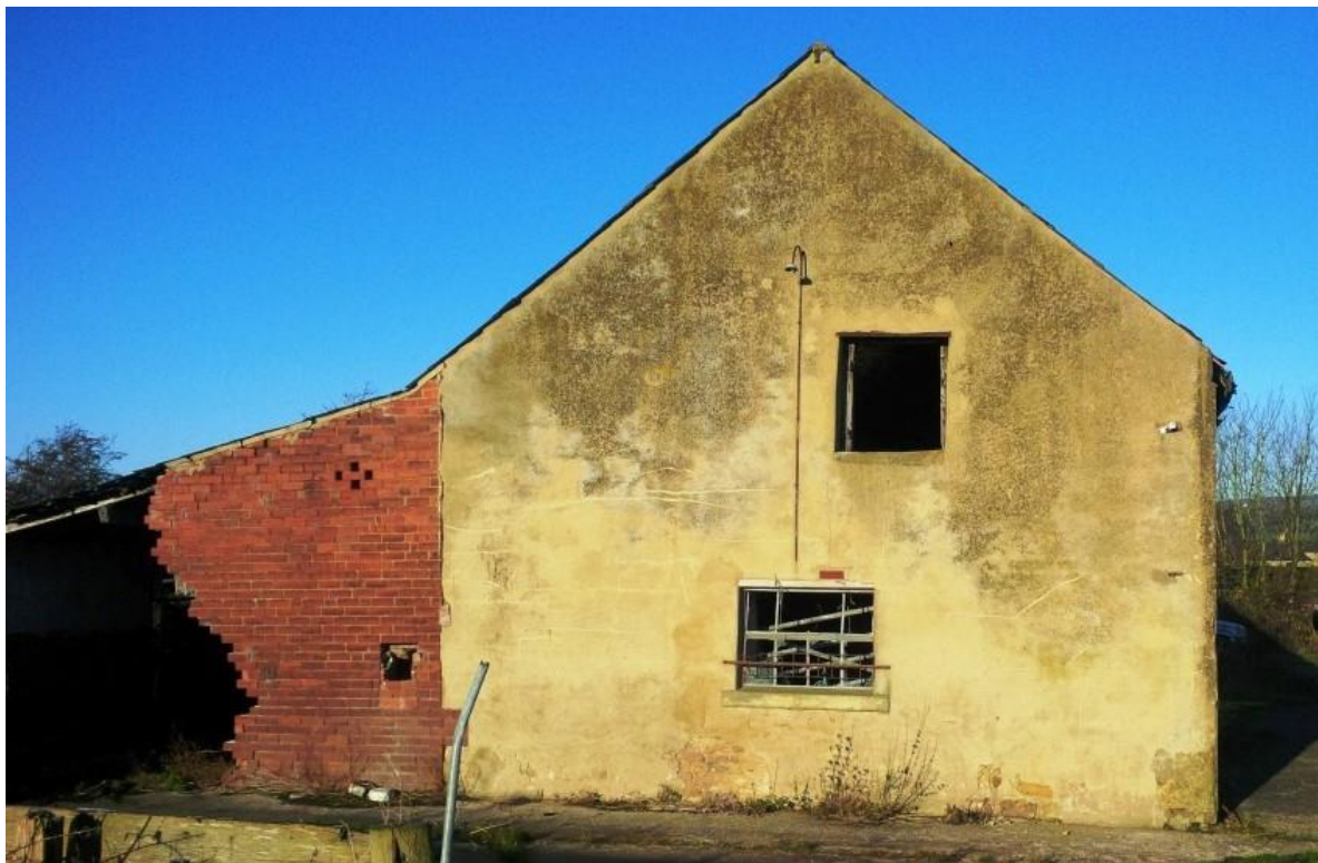
Figure 3. Southerly elevation showing added brick shippon and rendered original part
