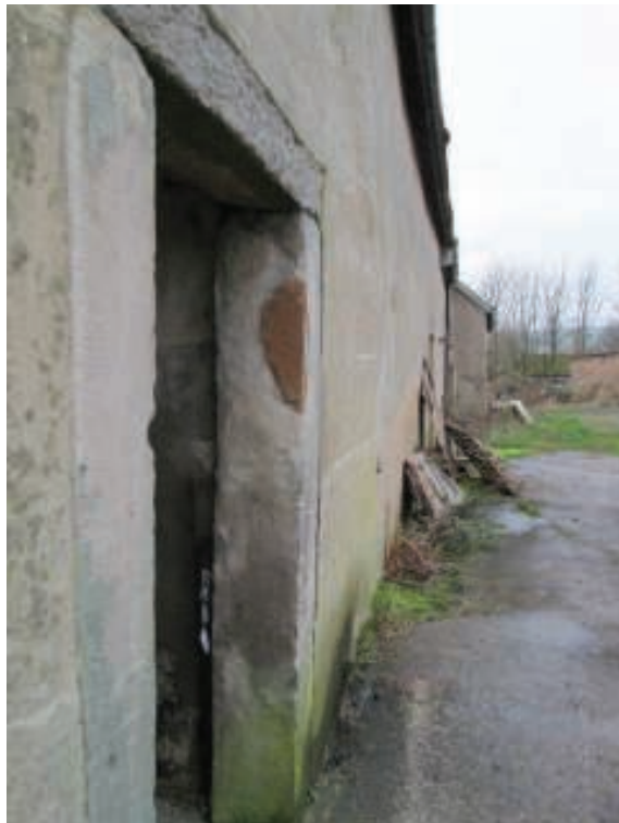
Photo 34 – Leaning Front Wall near Left-Hand Gable
