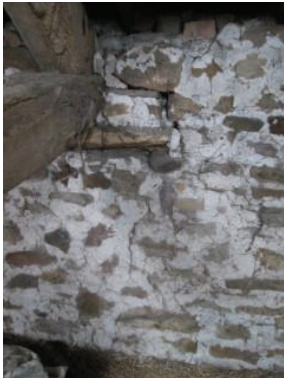
Photo 12 – Vertical Crack at Truss Bearing
