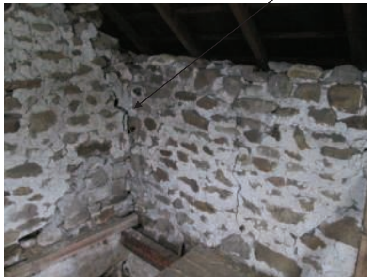
Photo 14 – Small Loft – Separation at Internal Wall / Front Wall Junction
