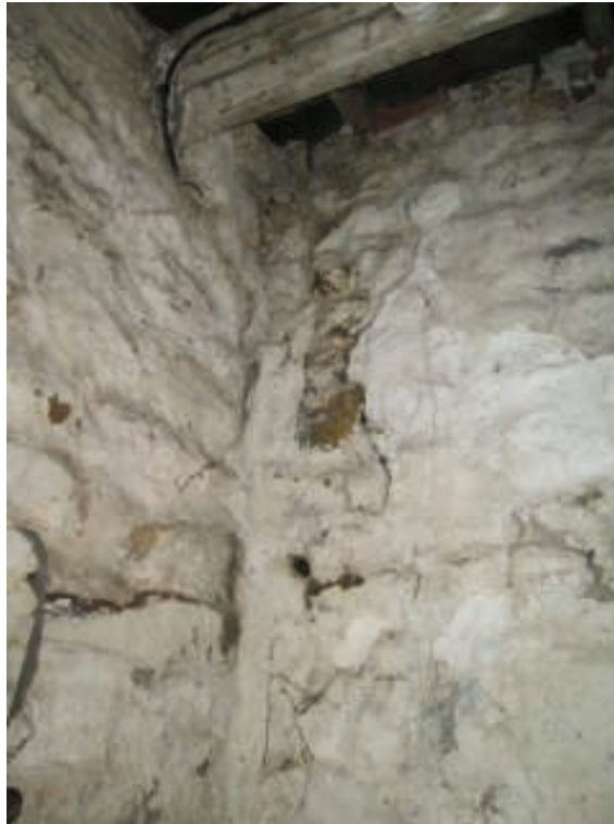
Photo 31 –Cracking in Rear Wall of Barn at Right-Hand Gable
