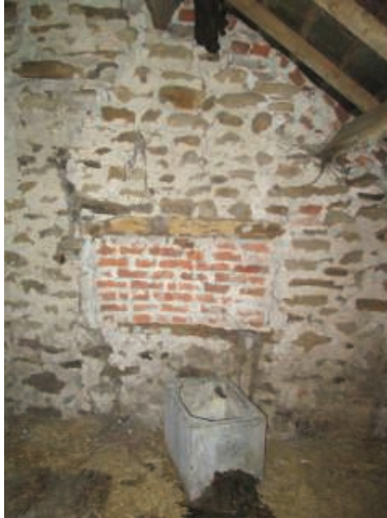
Photo 15 – Small Loft - Left Gable Wall – In-filled Opening
