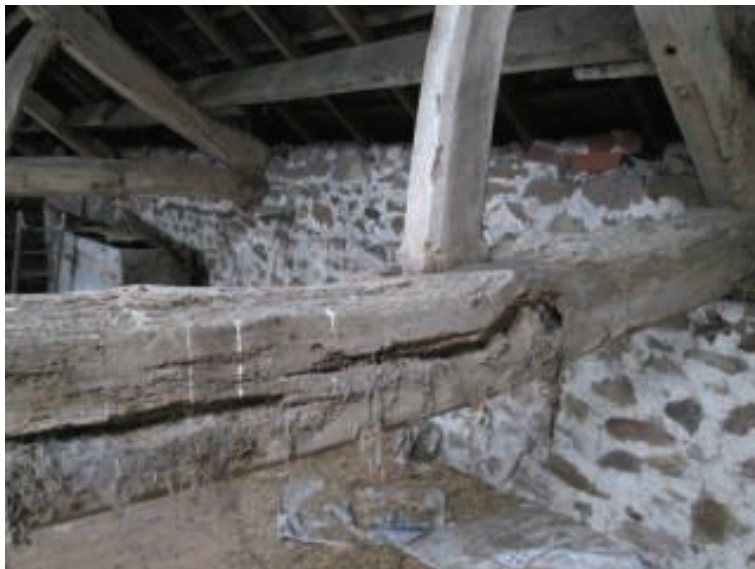
Photo 6 – Insect Damaged and Split Truss Bottom Tie
