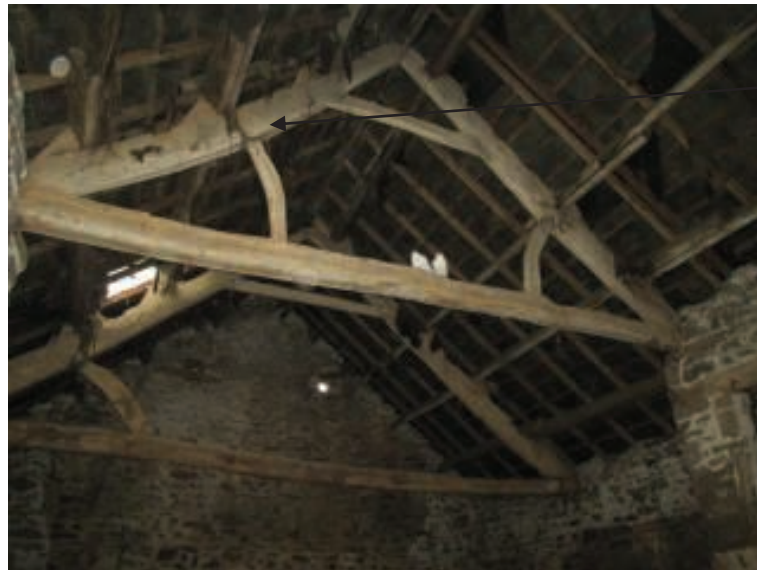
Photo 9 – Bowed Truss Principal Rafter.
