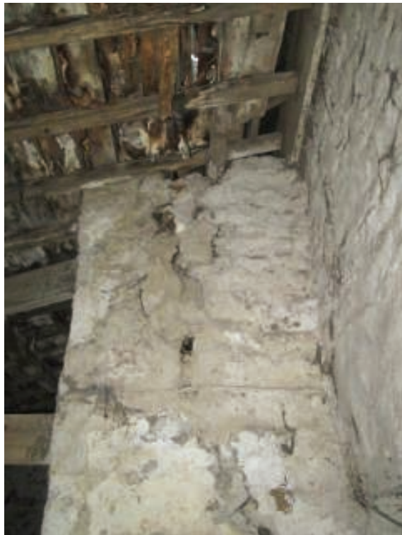
Photo 24 – Rear Wall of Barn – Vertical Crack (1)
