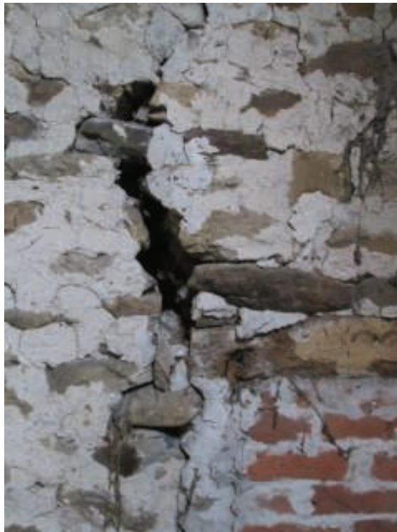
Photo 16 – Small Loft - Left Gable Wall – Wide Crack
