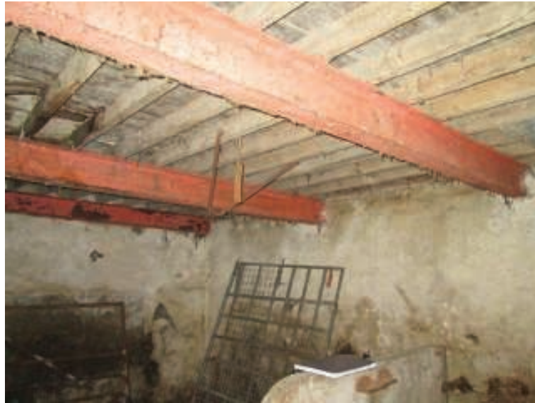
Photo 17 – Steel Beams Supporting Floor of Small Loft
