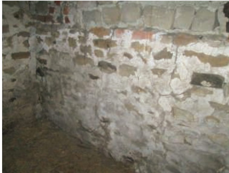
Photo 13 – Small Loft - Vertical Cracks in Rear Wall
