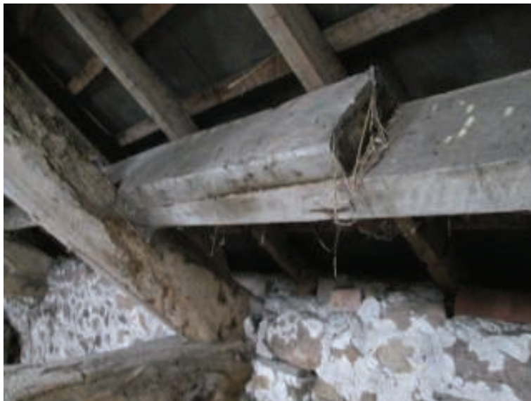
Photo 4 – Sawn Timber Rafters and Purlins
