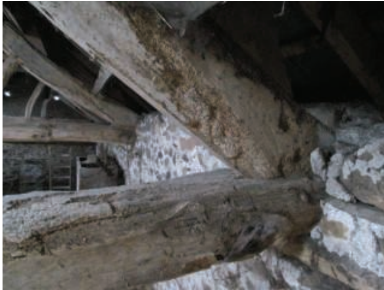
Photo 5 – Insect Decay at Truss Bearing
