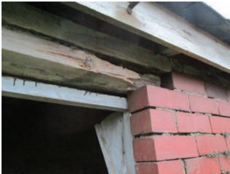
Photo 38 – Decayed Timber Lintels - Shippon
