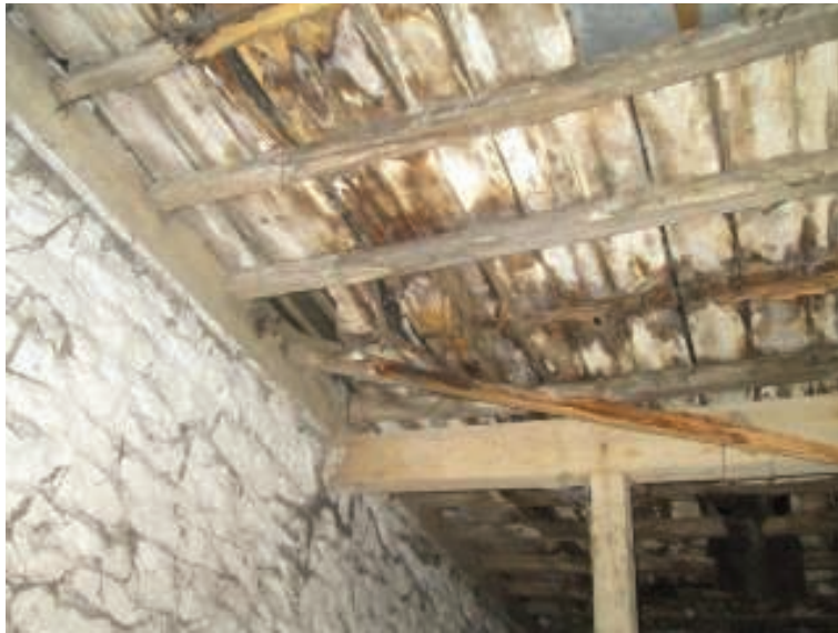
Photo 29 – Water Damage to Shippon Roof
