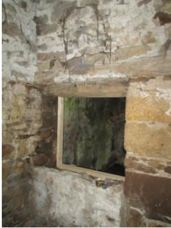
Photo 23 – Right-Hand gable Wall – Timber Lintels above Door / Window Opening
