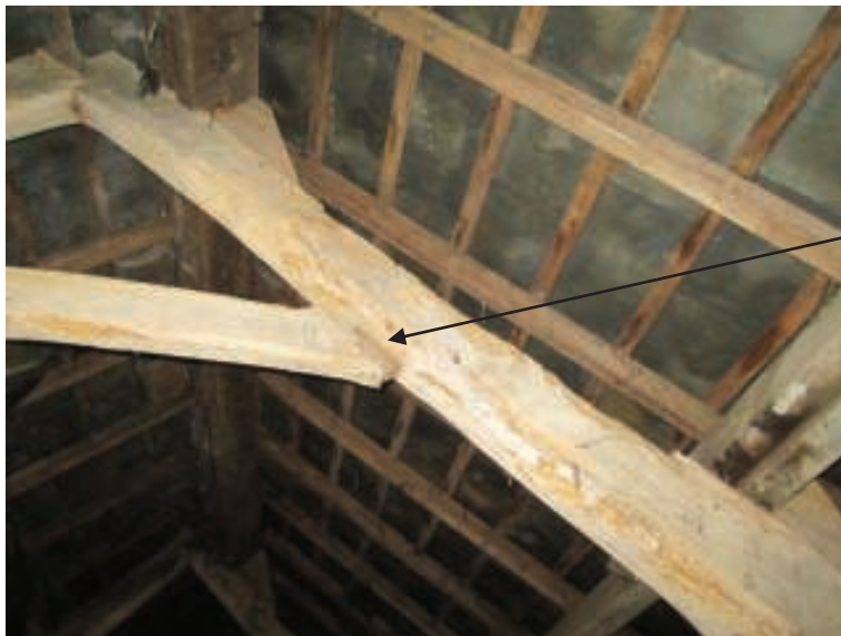
Photo 8 – Loose Truss Collar Tie
