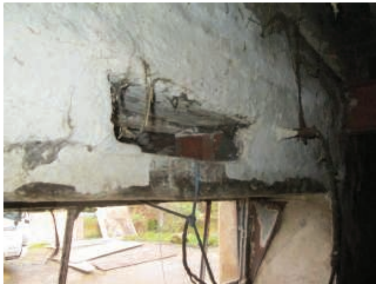
Photo 18 – Timber Lintel – Left Hand Gable Wall, Ground Floor
