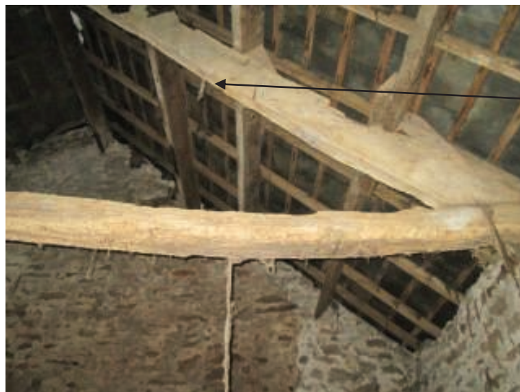
Photo 10 – Severe Bow and Insect Damage to Bottom Tie Beam. Missing Strut
