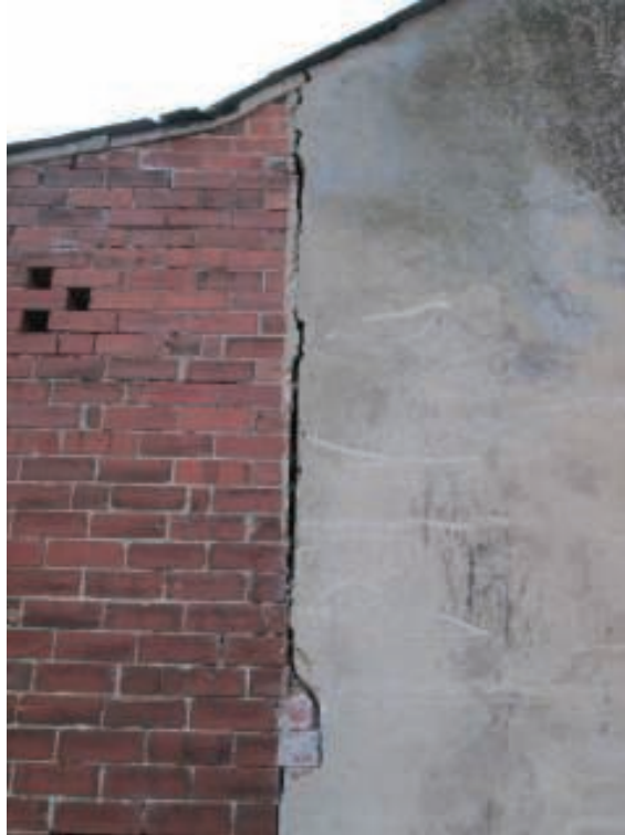
Photo 39 – Gap between Shippon and Barn - Left-Hand Gable Wall
