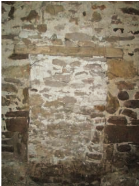
Photo 22 – Right-Hand Gable Wall – In-filled Door Opening
