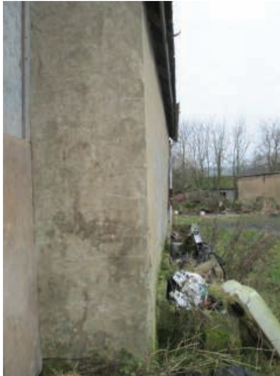
Photo 35 – Leaning Front Wall at Entrance Door
