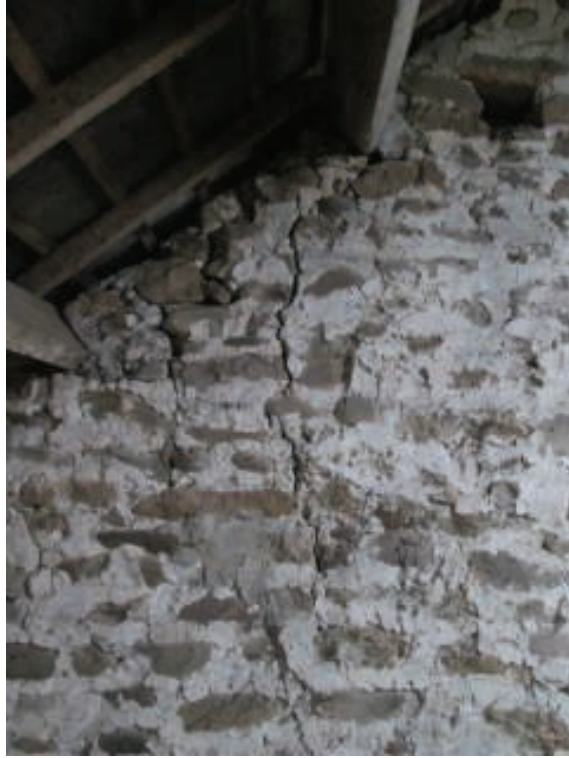
Photo 11 – Vertical Crack in Central Wall
