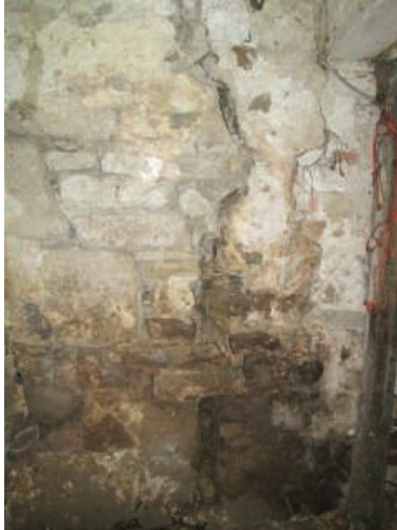
Photo 25 – Rear Wall of Barn – Vertical Crack (2)
