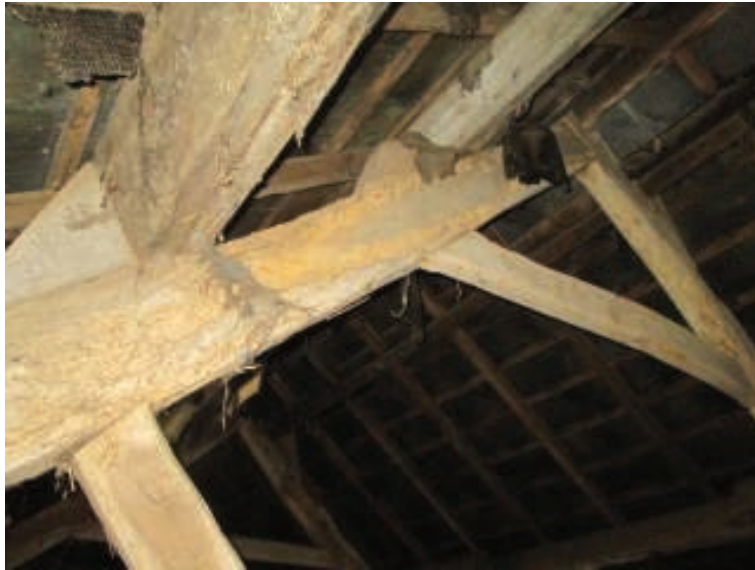
Photo 7 – Insect-Damaged Truss Principal Rafter
