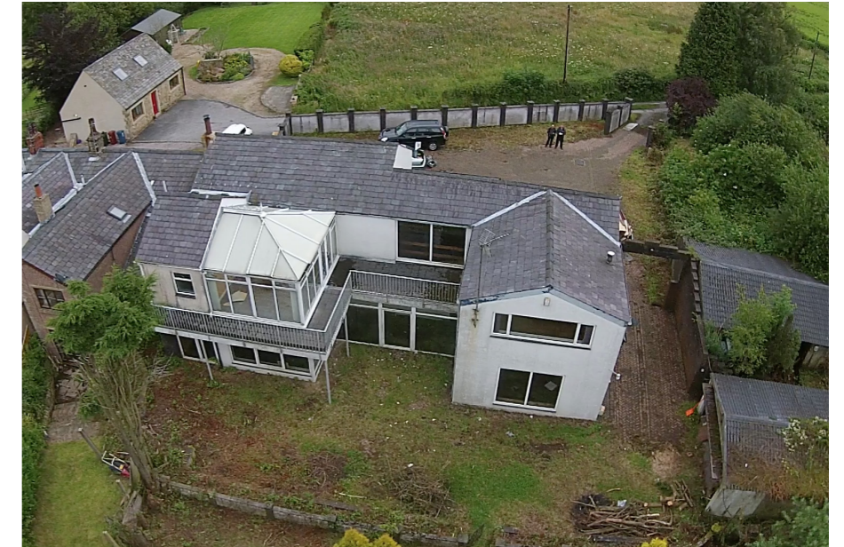
Aerial view of existing
