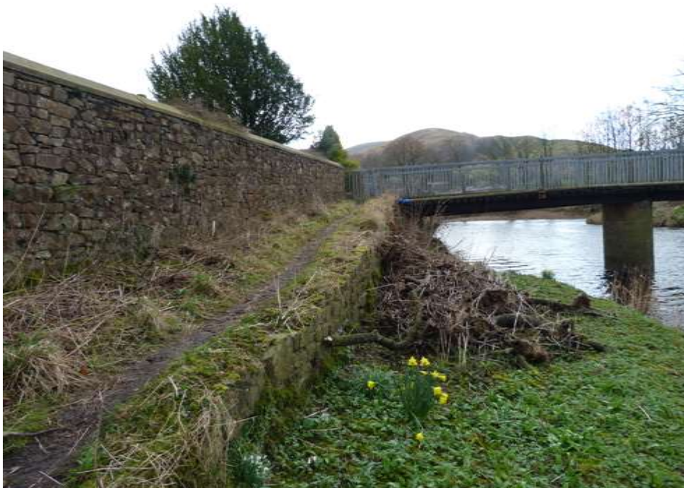
Photograph 4 – Wall at Thorneyholme Bridge over River Hodder at northwest corner of the site
