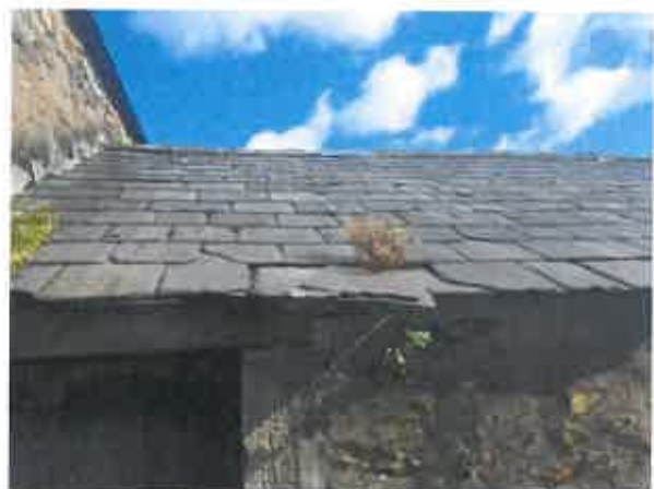
PL2 (Left) and PL3 (Right) showing cracked, chipped and dislodged slates along with vegetation growth.
