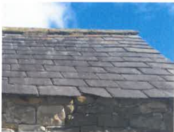
PL2 (Left) and PL3 (Right) showing cracked, chipped and dislodged slates along with vegetation growth.
