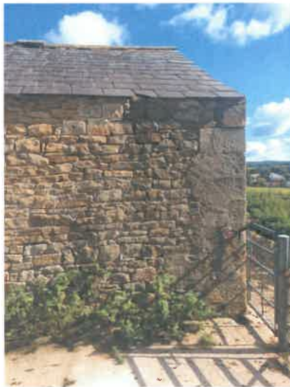
PL35 (Left) shows mortar repairs to stone joints and significant plant / weed growth to base of wall. PL36 (Right) showing mortar patch repairs, mortar degradation and plant / weed growth.
