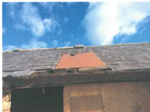
PL6 (Left) and PL7 (Right) showing cracked, chipped and dislodged slates with ad-hoc roofing repair. Degradation and missing mortar pointing noted to roof verges.
