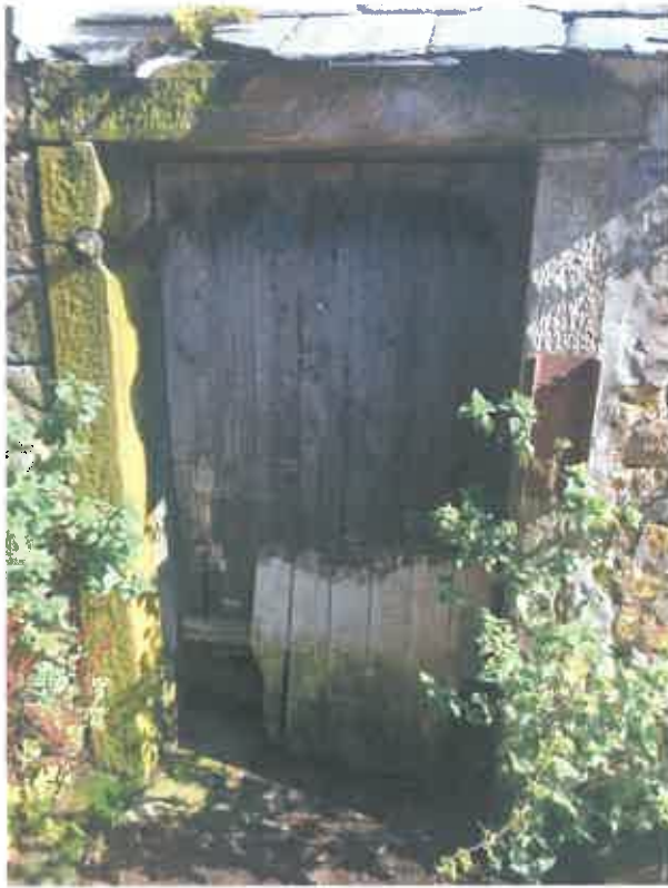
PL46 (Left) and PL47 (Right) showing dilapidated and damaged external doors.
