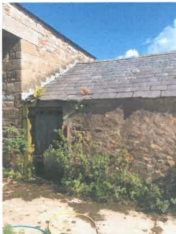
PL35 (Left) shows mortar repairs to stone joints and significant plant / weed growth to base of wall. PL36 (Right) showing mortar patch repairs, mortar degradation and plant / weed growth.
