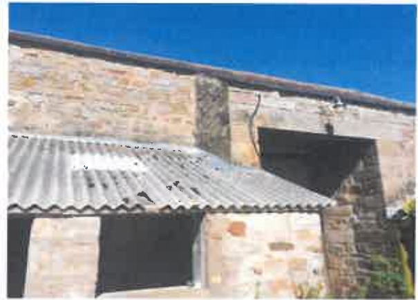
PL8 (Left) and PL9 (Right) showing the condition of the asbestos roof covering and the section of dislodged lead flashing (this particular area is to be demolished).
