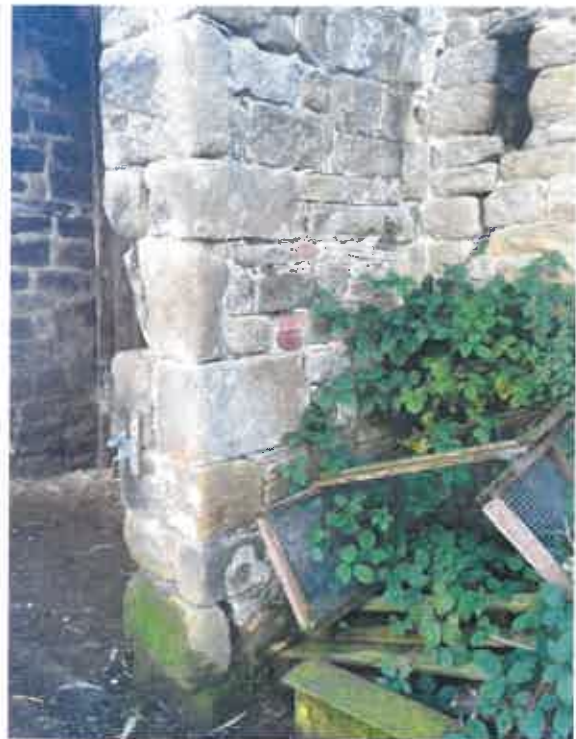
PL21 (Left) showing mortar crack to right hand side of stone lintel to barn entrance. PL22 (Right) showing condition of stonework and degradation to base of wall.
