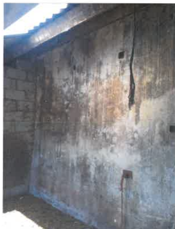
PL40 (Left) shows wall cracking to the internal face of the east gable wall within the north section of the barn and is in the same location as the external wall cracking. Minor isolated crack stitching / lateral restraint ties potentially required at this point. PL41 (Right) shows soiling and staining to internal walls.
