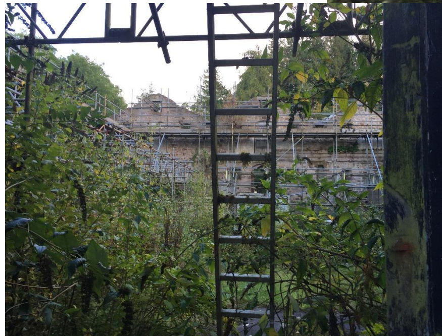
The Mill - existing condition
