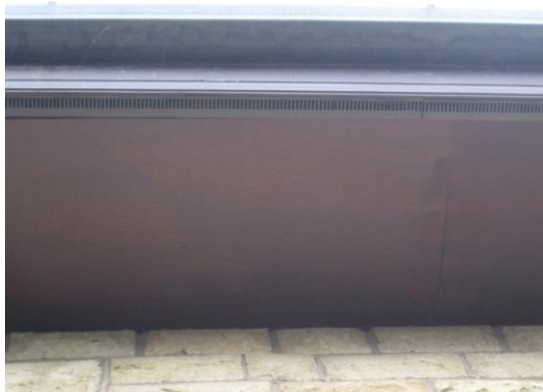
Figure 5: Air vent on edge of soffit
