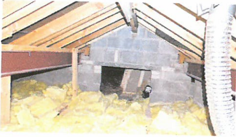
Figure 8: roof void 'A'
