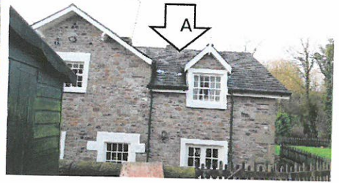
Figure 4: side elevation and roof void 'A'
