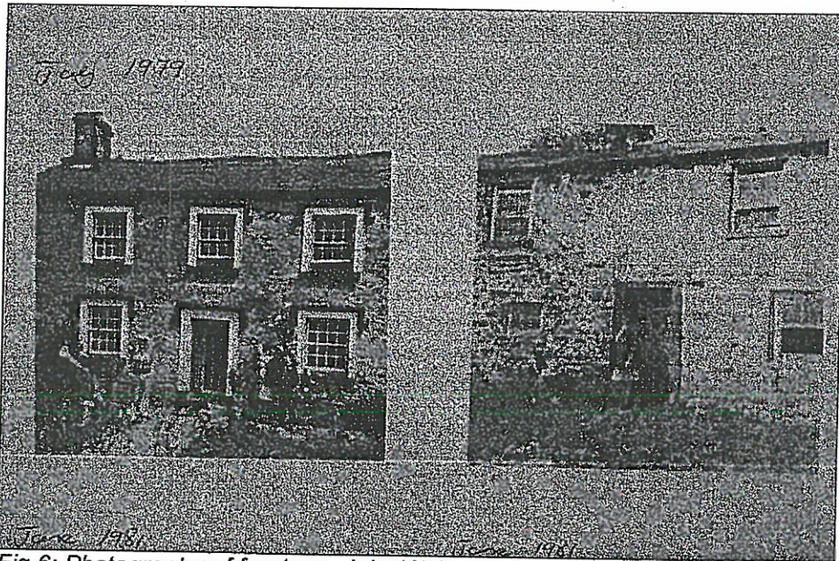
Fig. 6: Photographs of frontage, July 1979
