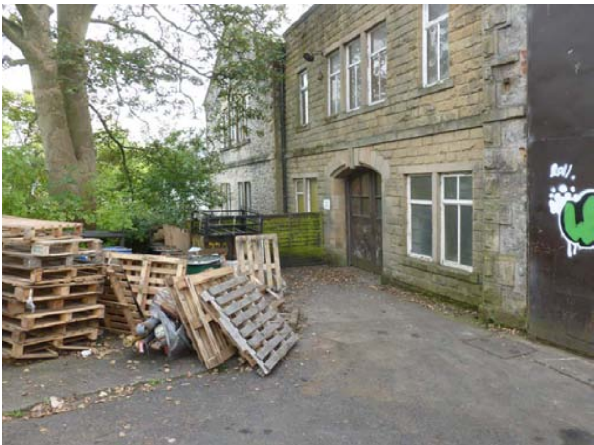
Photo 6 – S & Central building from NE yard, looking S.
