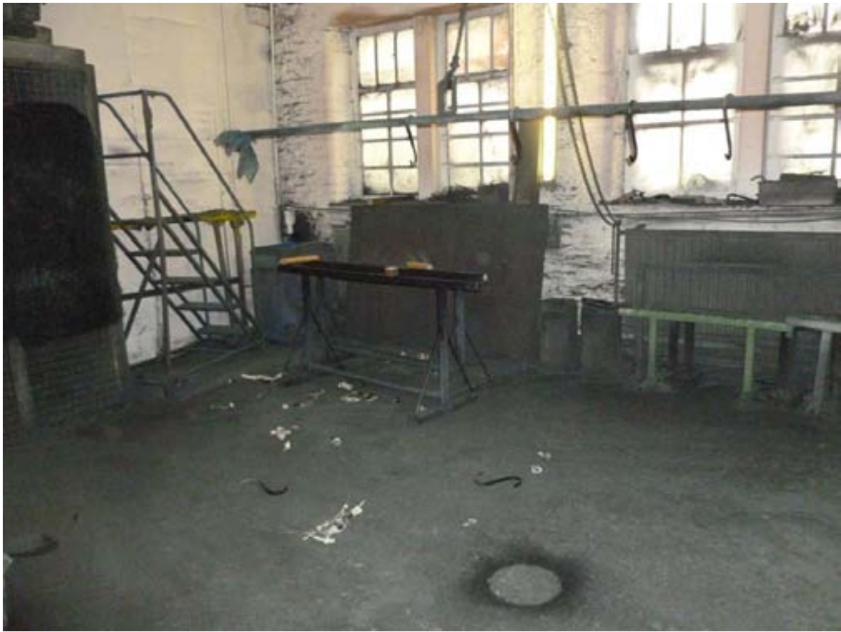
Photo 17 – Internals of paint shop in W area of Central Building, looking W.
