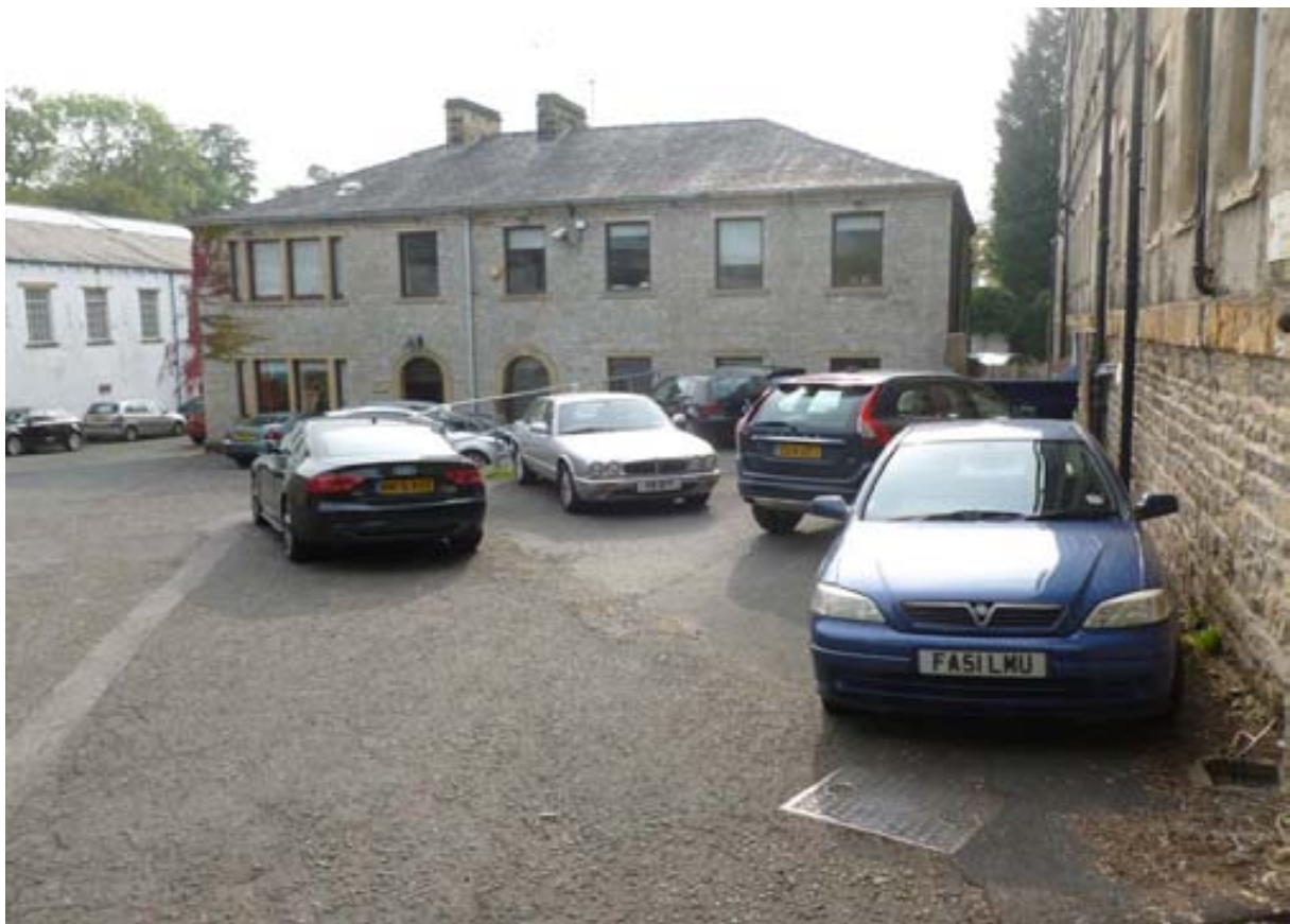
Photo 2 –Lower southern car park, looking W.
