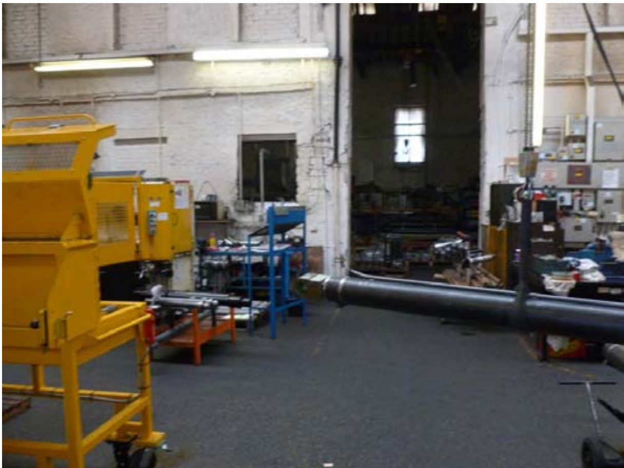
Photo 16 – Internals of Central building with concrete floors, looking N.
