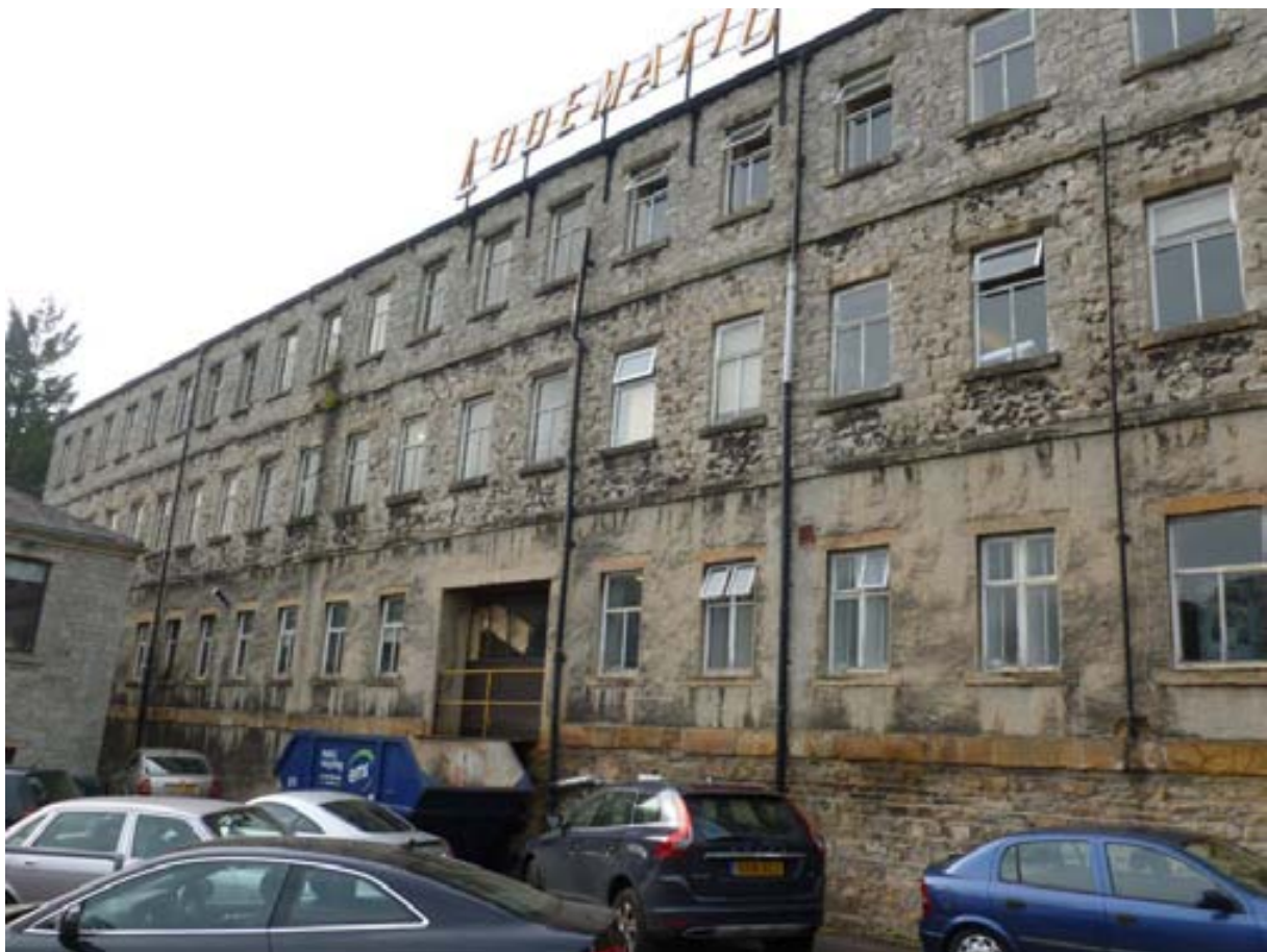
Photo 1 – Lodematic (southern) Building, looking NW.
