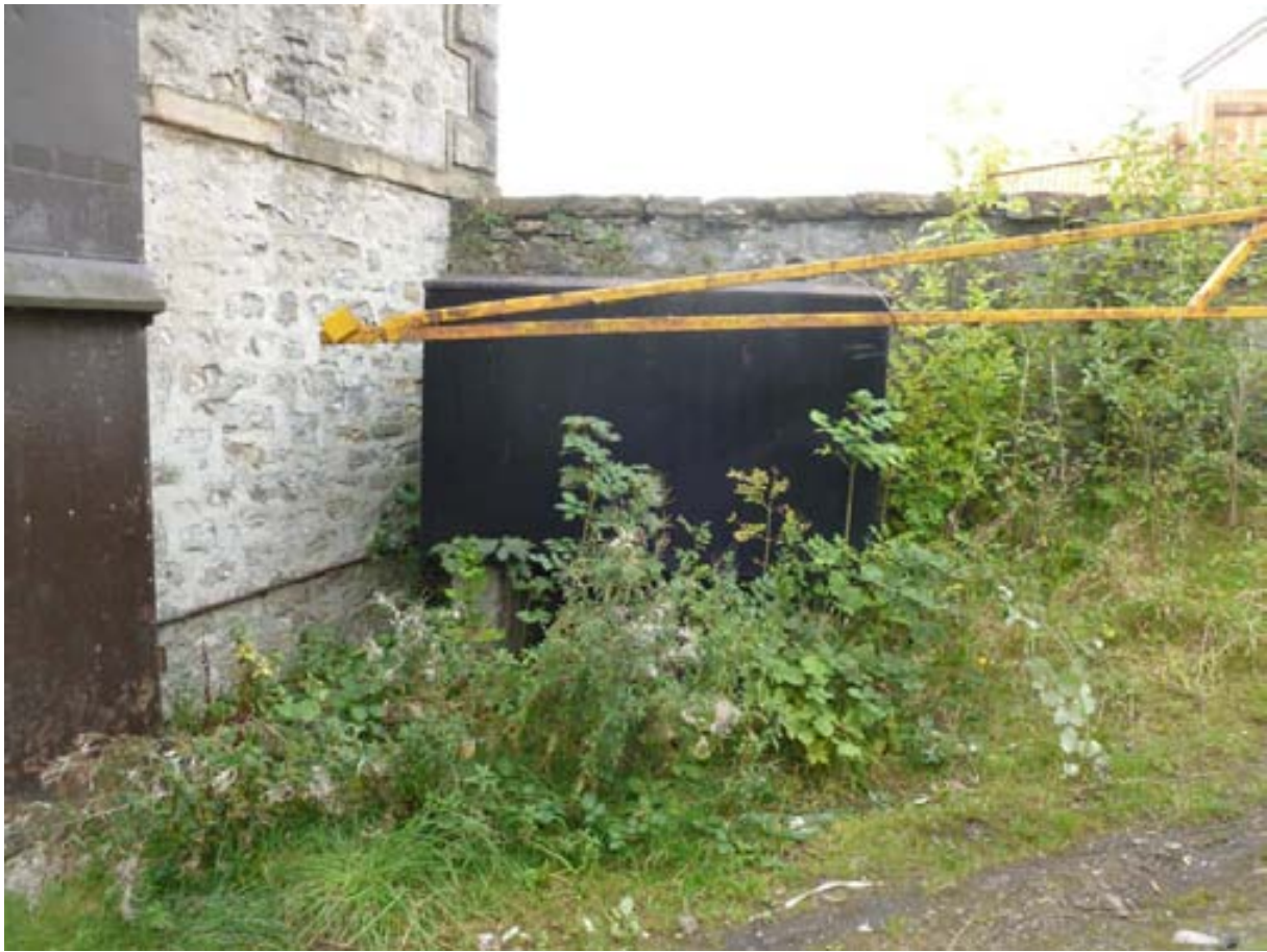
Photo 7 – Disused tank outside NE corner of main buildings, looking N.
