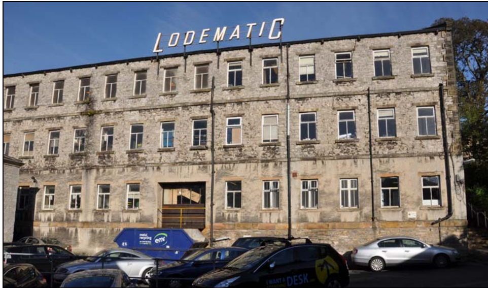
Photo 1: Building 1, main block
