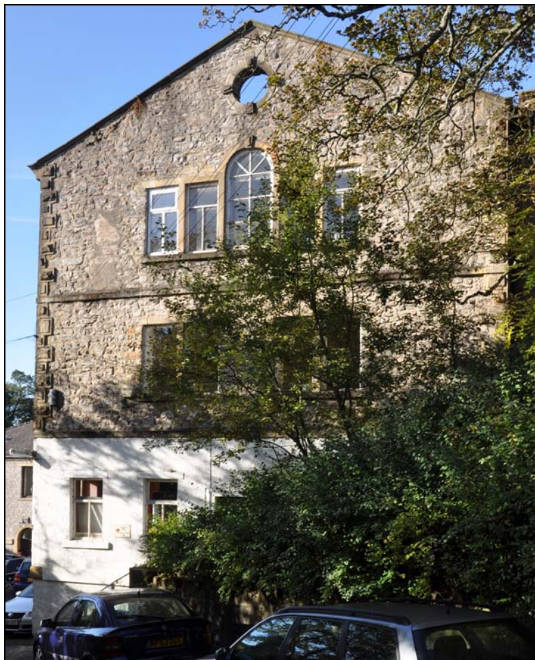
Photo 2: Building 1, north-east gable
