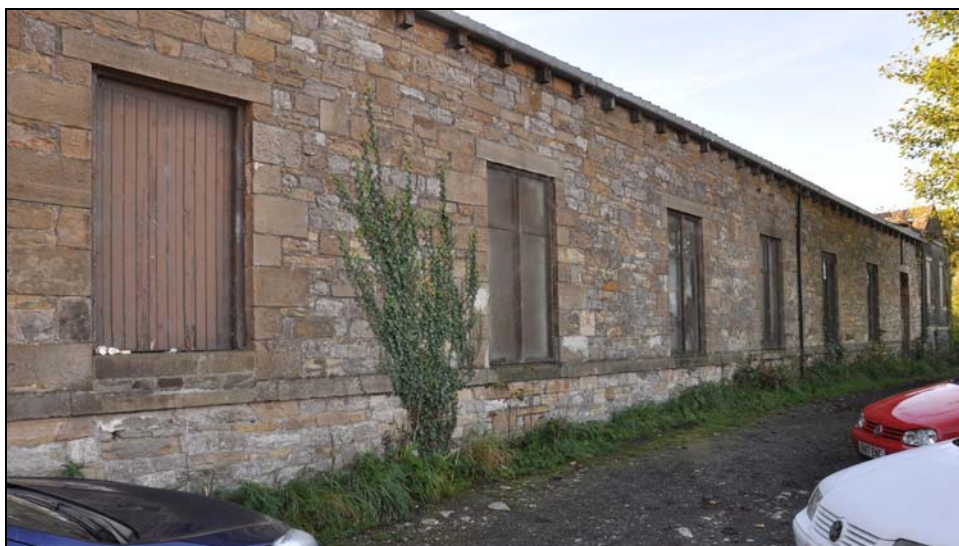
Photo 6: Building 2, north-west elevation
