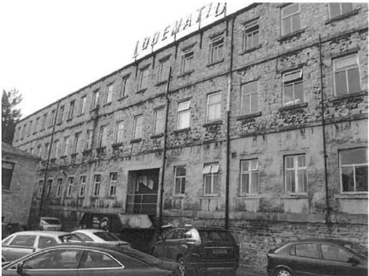
Photo 1 – Lodematic (southern) Building, looking NW.
