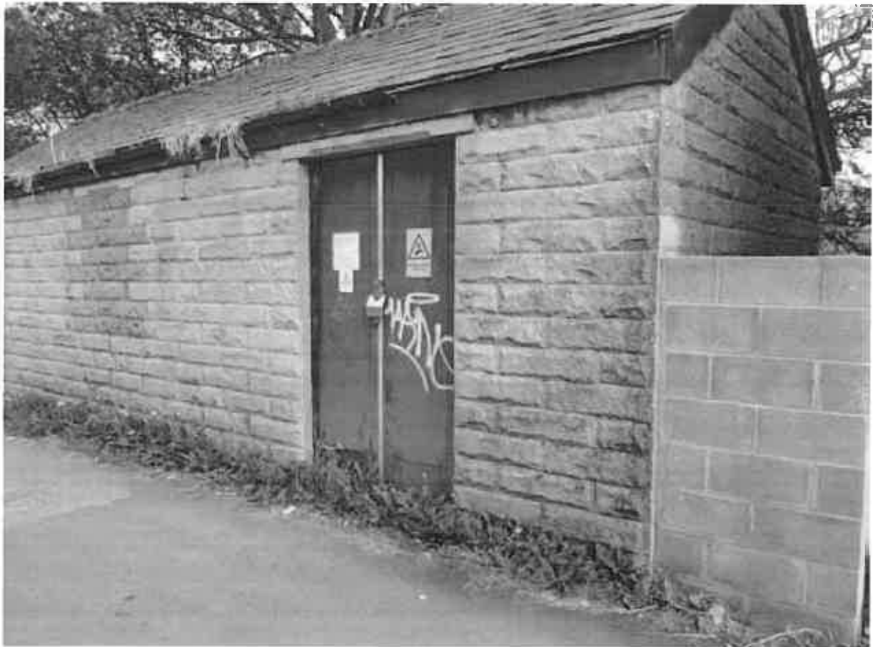
Photo 10 – Electrical sub-station adjacent to NE boundary of site, looking SE.
