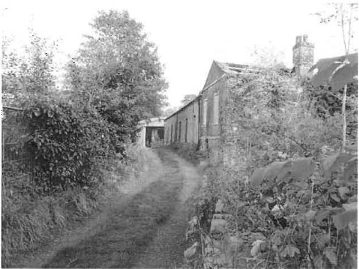
Photo 5 – Track running along N boundary of site, looking E.
