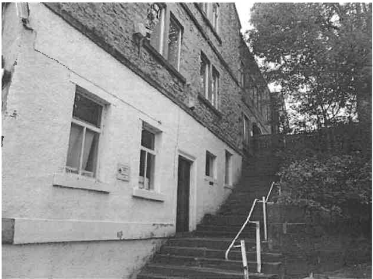
Photo 3 – Eastern edge of buildings, with steps leading up the steep slope, looking NW.
