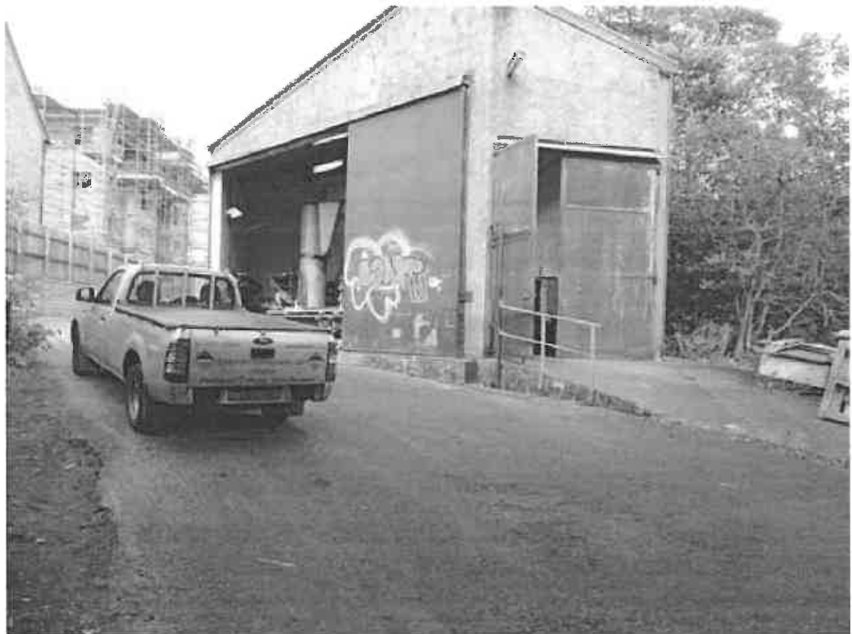
Photo 8 – Smaller detached building within NE corner of site, looking NE.
