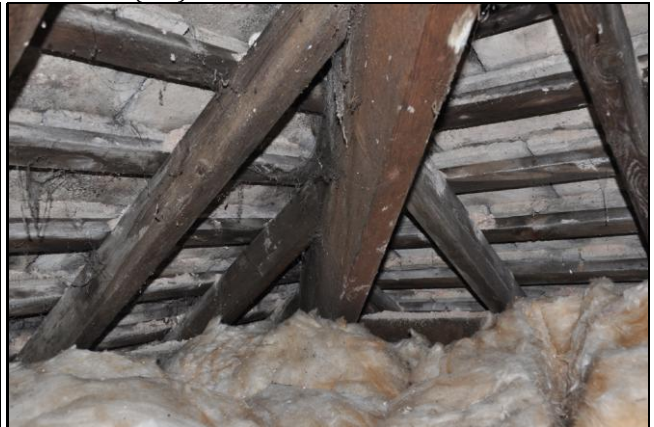
View of small, shallow, unlined roof void(rhs)
