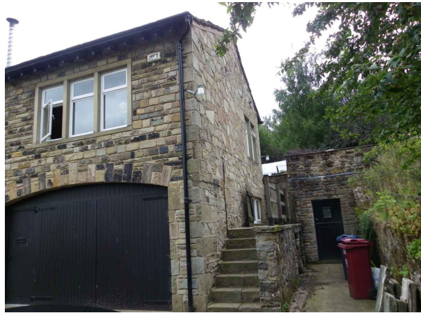
detail view at north corner
