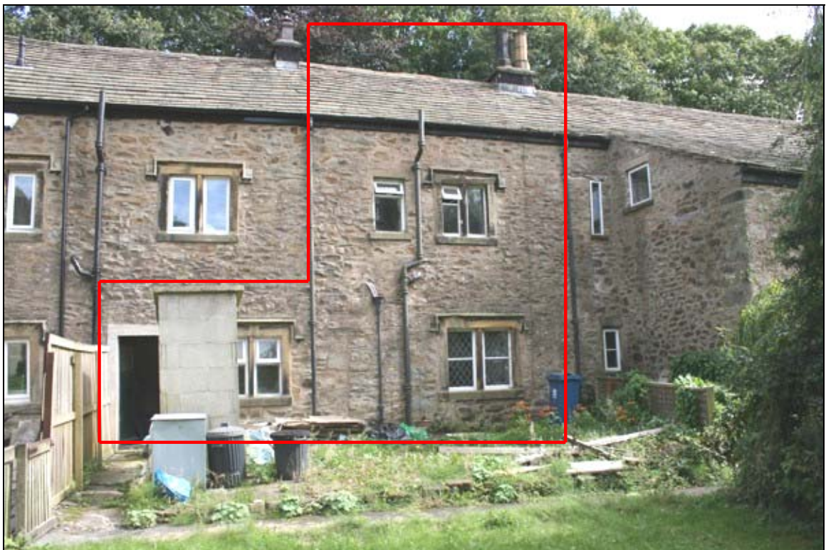
8. General view of rear, showing extent of Number 2; ground floor entrance to kitchen on left
