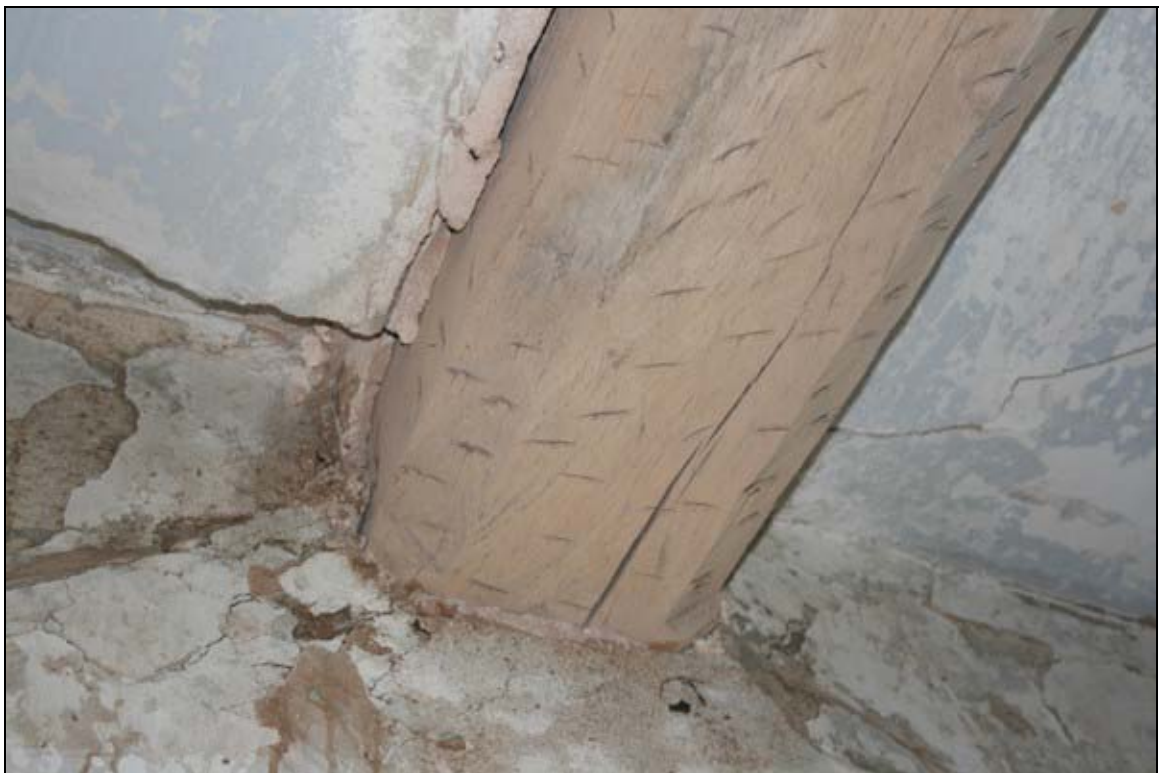
21. Chamfered first floor beam (tiebeam of roof truss)
