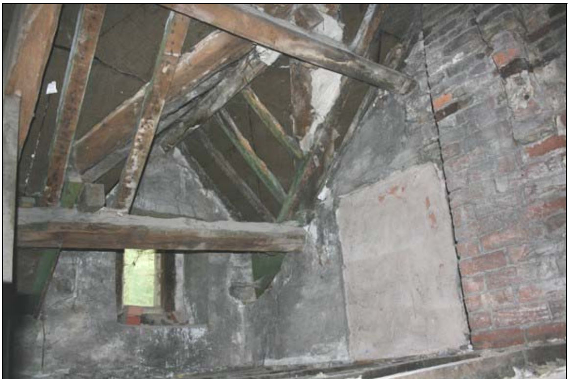
23. Blocked doorway to Number 4 in attic, left of flue
