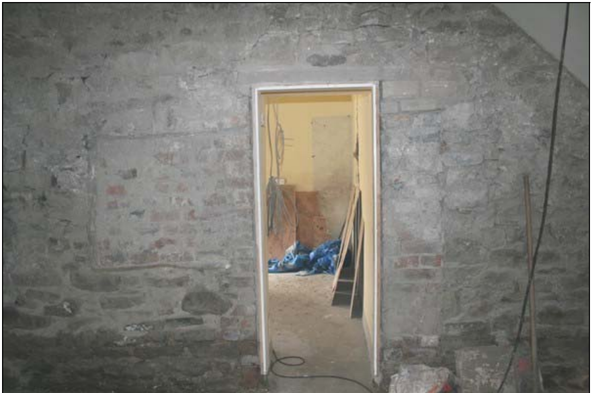
16. Outline of blocked window in crosswall pierced by later inserted door
