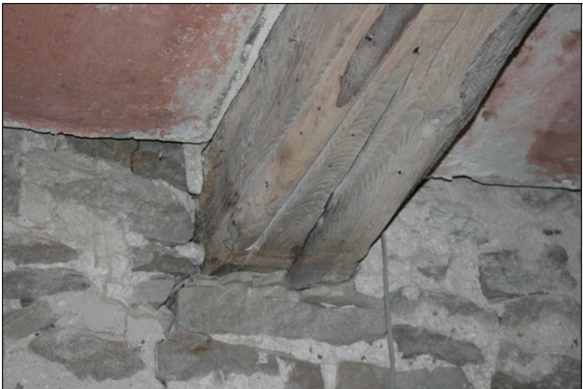
13. Stopped roll- moulded beam on ground floor
