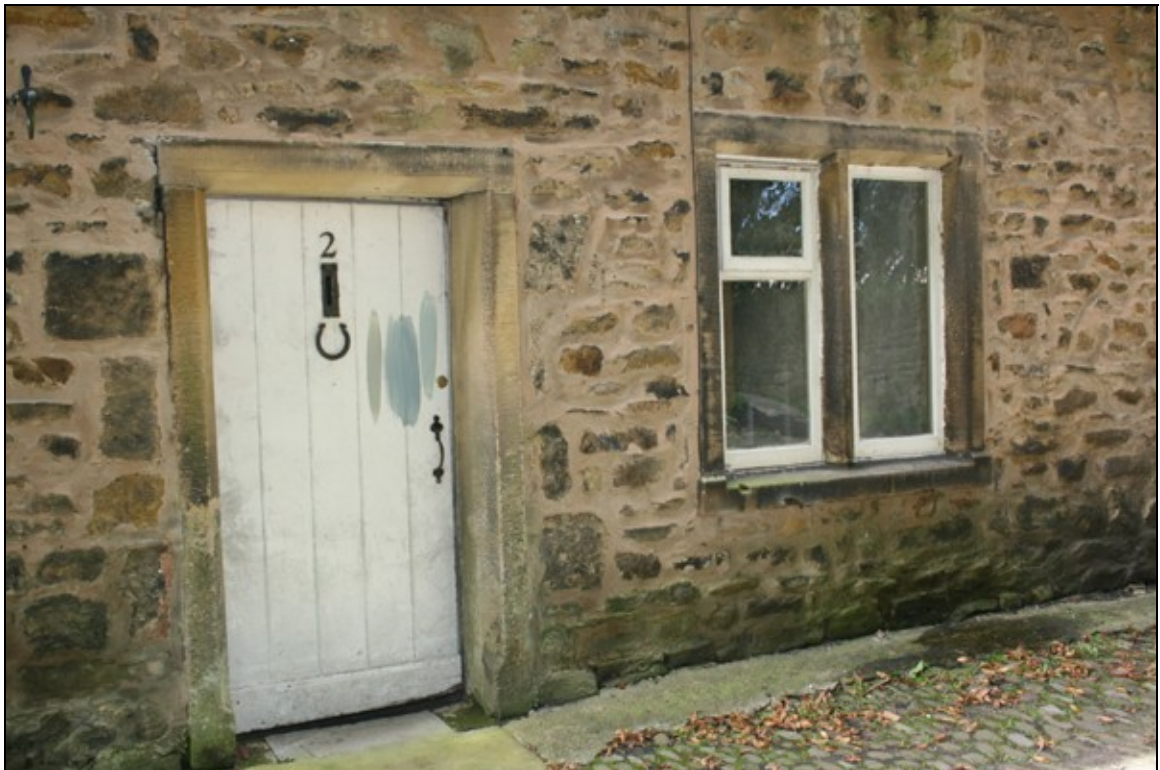
6. Detail of entrance showing earlier long-and-short quoins on either side of 19 th century surround
