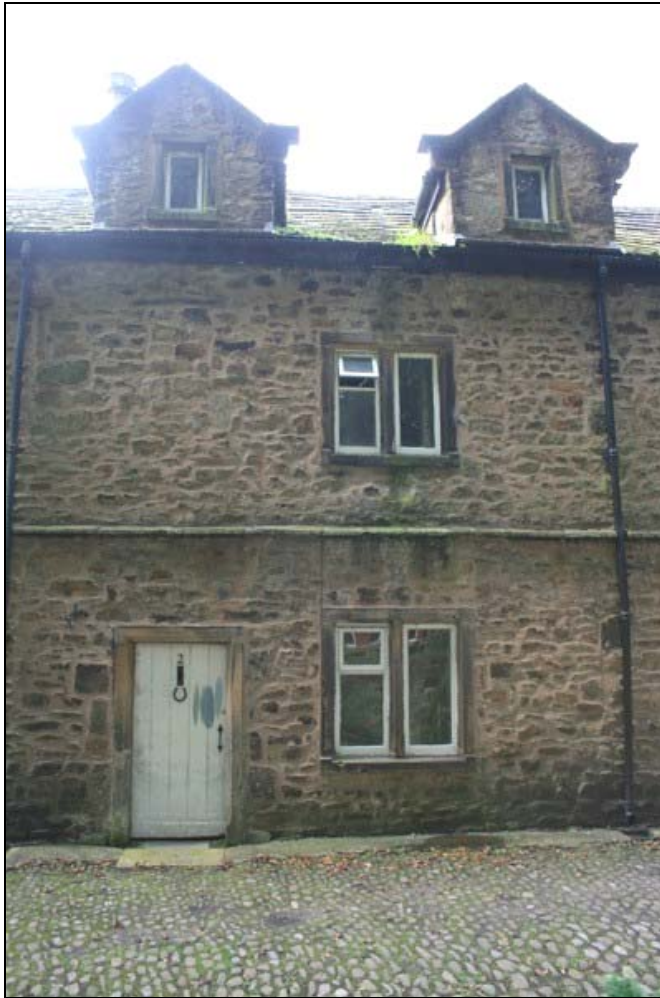
5. Front elevation of 2 Abbeycroft, showing evidence of quoins at right end and blocked windows on first floor
