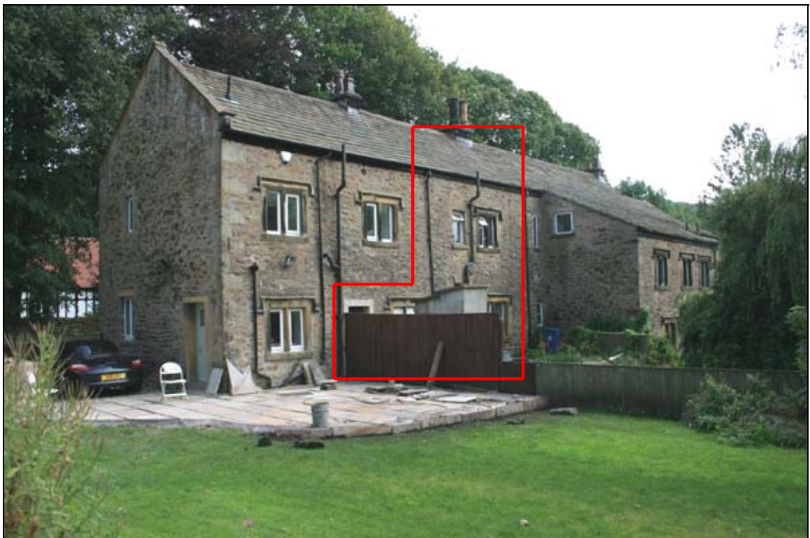
3. View of the rear of Abbeycroft, Number 2 indicated, showing L-shaped arrangement
