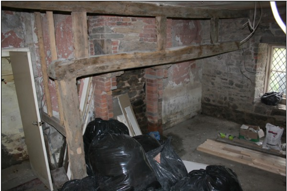
11. Interior of ground floor living room, showing skeletal firehood structure
