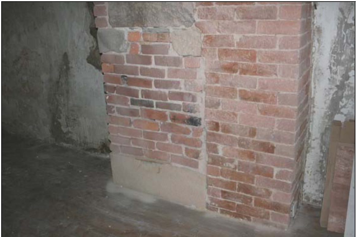
20. Blocked first floor hearth
