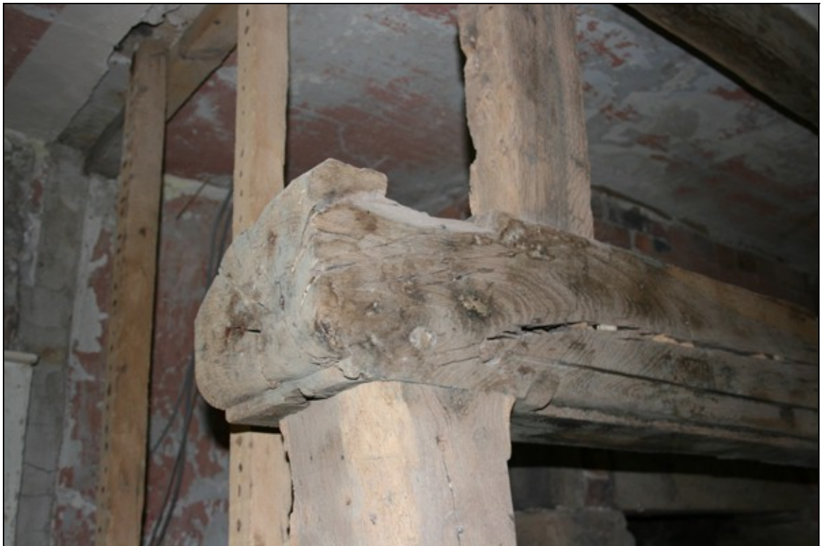
12. Detail of chamfered heck post supporting bressumer
