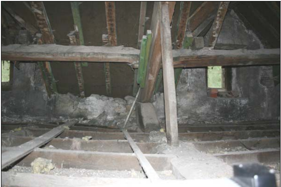
22. Part of roof truss showing angle strut and lower purlin
