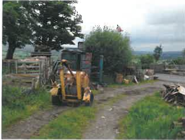
Site container and storage compound
