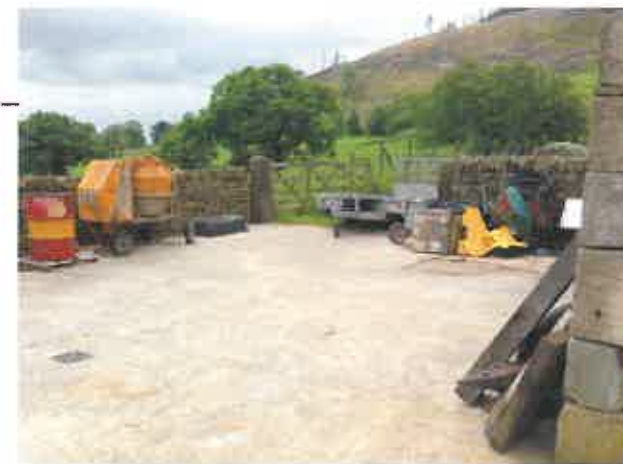
Plant holding and repair area
