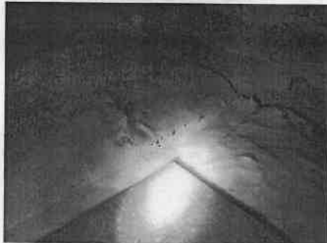
Plate 4: Collections of droppings were found directly on the insulation within the loft.
