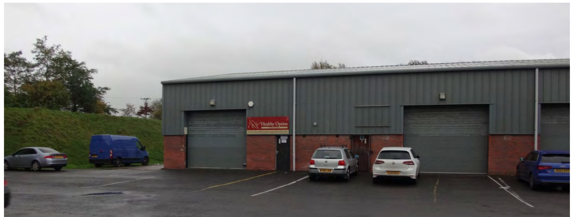
View from the site looking to the East.
