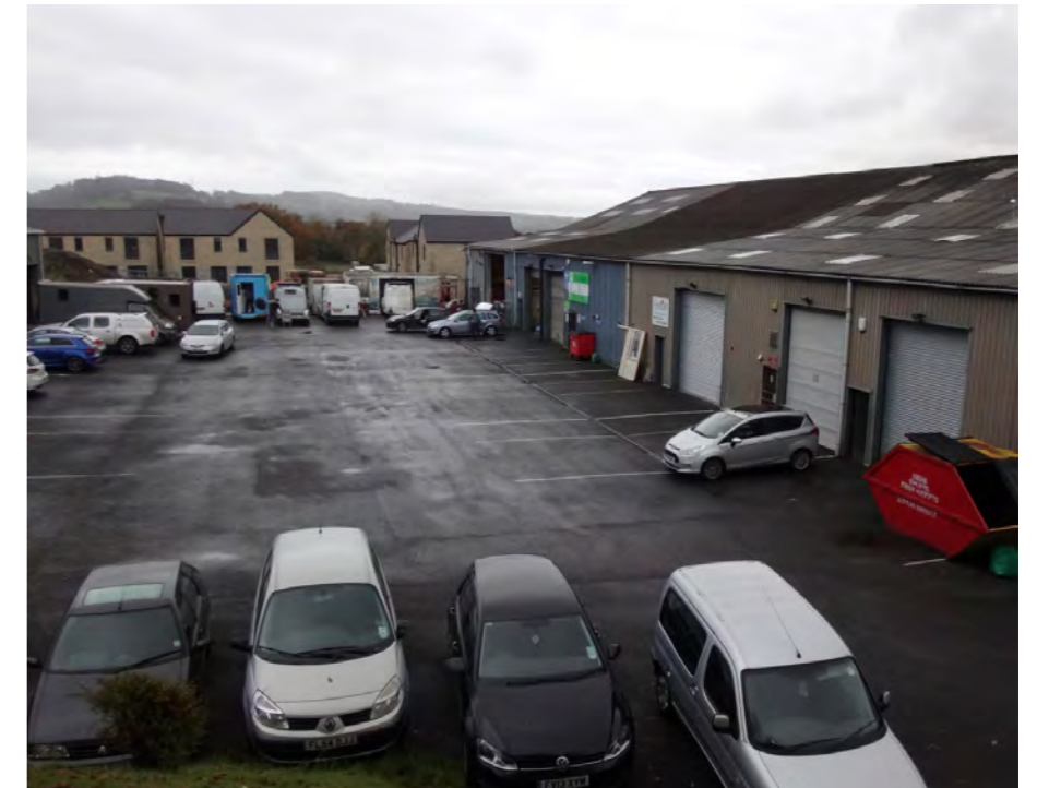
View from the Northern boundary looking South West
