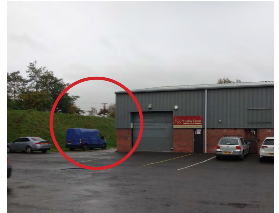
Existing unit to be extended, Whalley Industrial Park
