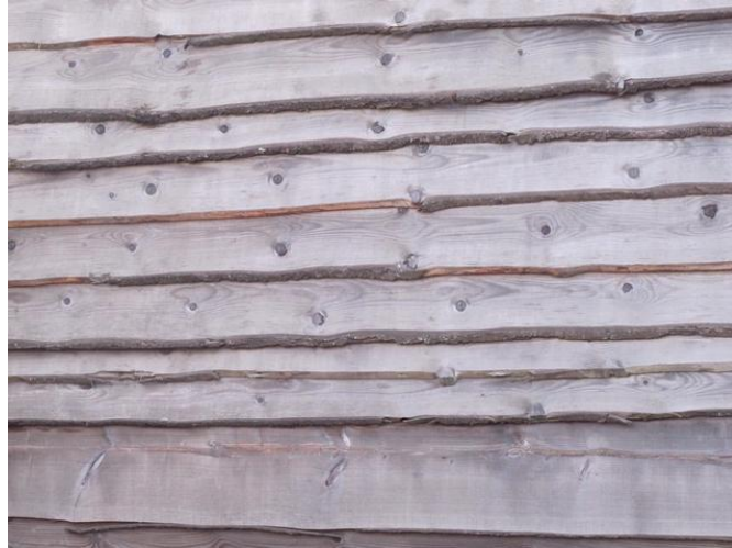
Photograph 3 – Waney edge larch cladding
