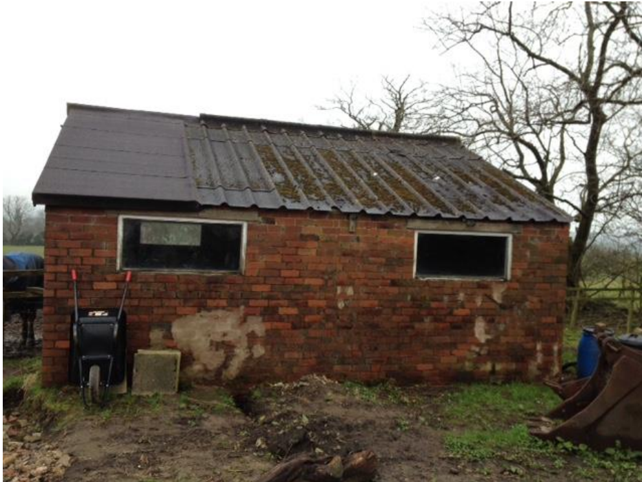
Photograph 1 – Building to be converted
