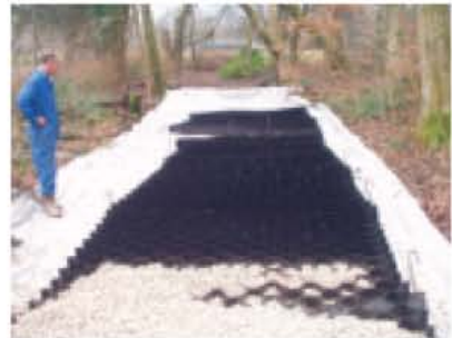
Installation of the CellWeb™ system.
