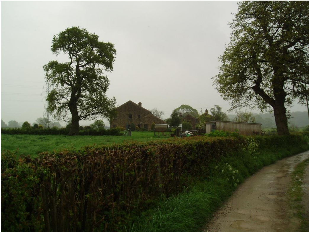
7 Outbuilding to be demolished
