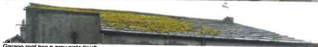
Garage roof has a grey slate finish.
