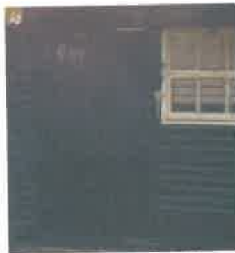
The stables are timber boarding.
