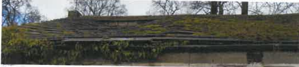
Stable roof - corrugated asbestos sheet with clear plastic roof lights
