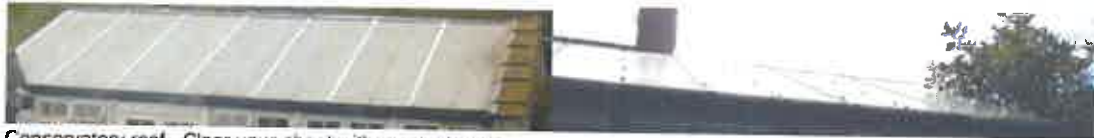
Conservatory roof - Clear upvc sheet with verge stones
