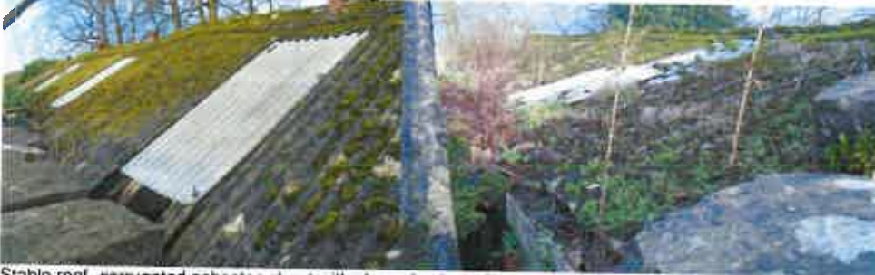
Stable roof - corrugated asbestos sheet with clear plastic roof lights
