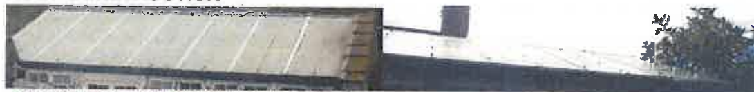
Conservatory roof - Clear upvc sheet with verge stones
