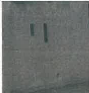
The garage walls are rough cast render.
