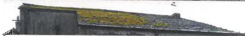
Garage roof has a grey slate finish.
