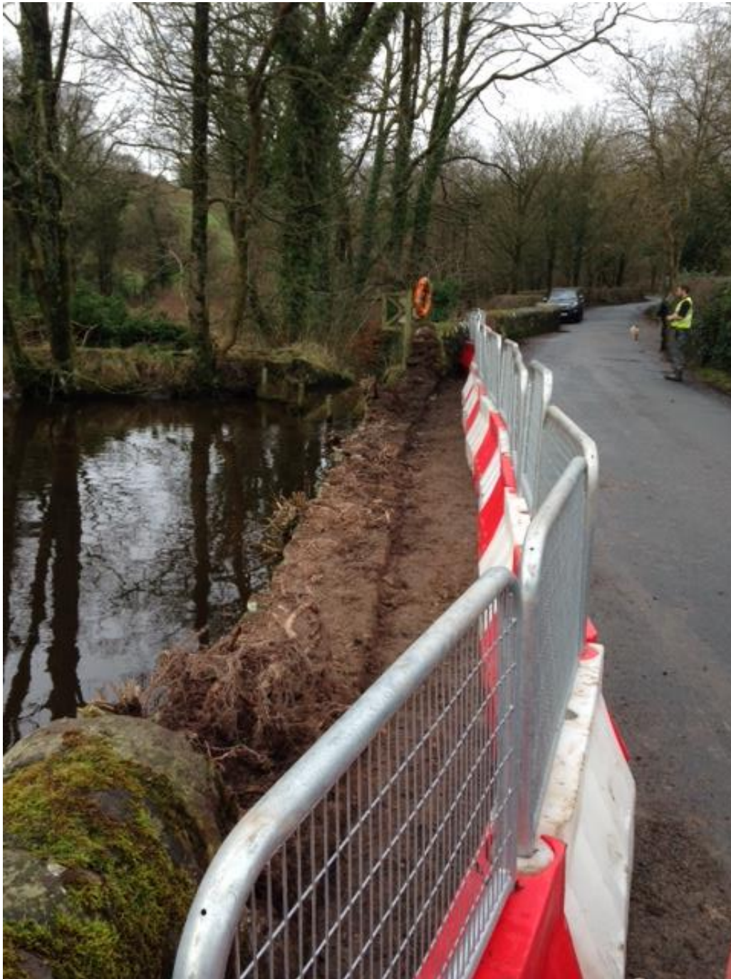
Photograph 15: Location of Dismantled Mill Pond Wall
