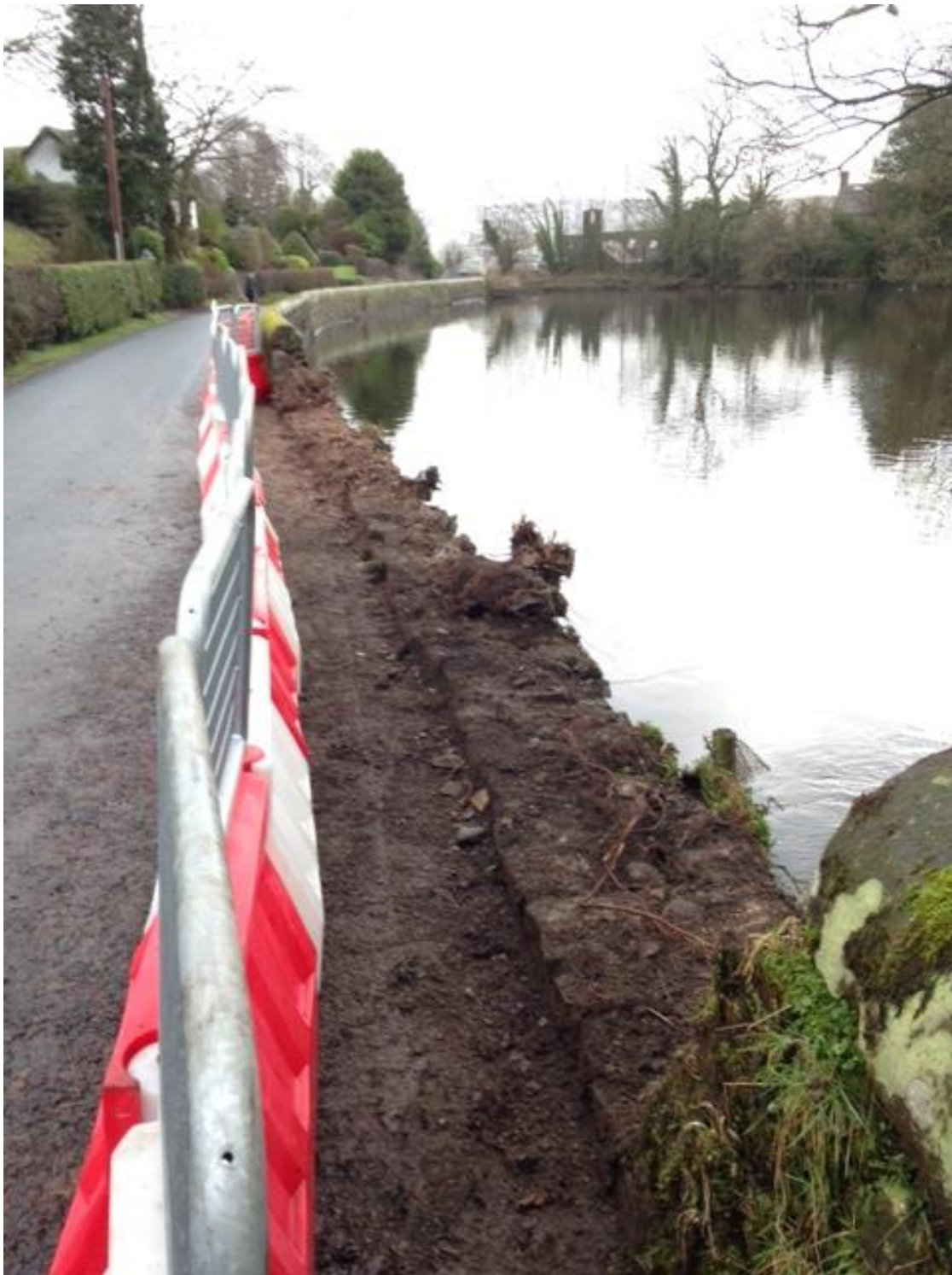
Photograph 16: Location of Dismantled Mill Pond Wall
