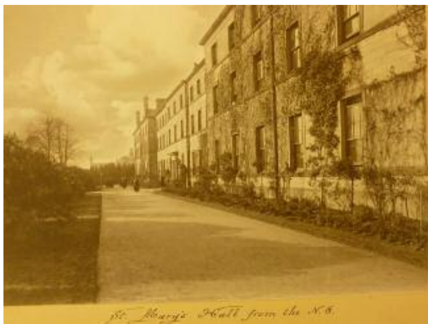
Fig.2: St Mary's Hall and the terrace in c1900 (Stonyhurst Archive)
