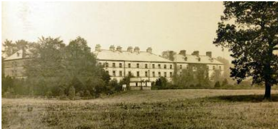
Fig.5: St Mary's from the south-west in c1900 (Stonyhurst Archive)
