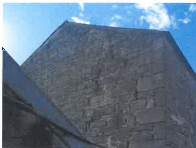
PL25 (Left) showing condition of the east elevation gable wall with degraded mortar and patch repairs. PL26 (Right) showing cracking to east elevation gable wall.
