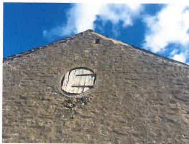
PL48 (left) showing dilapidated window frame with wire mesh infill. PL49 (Right) showing poor condition of pitching hole door and rusting hinges.
