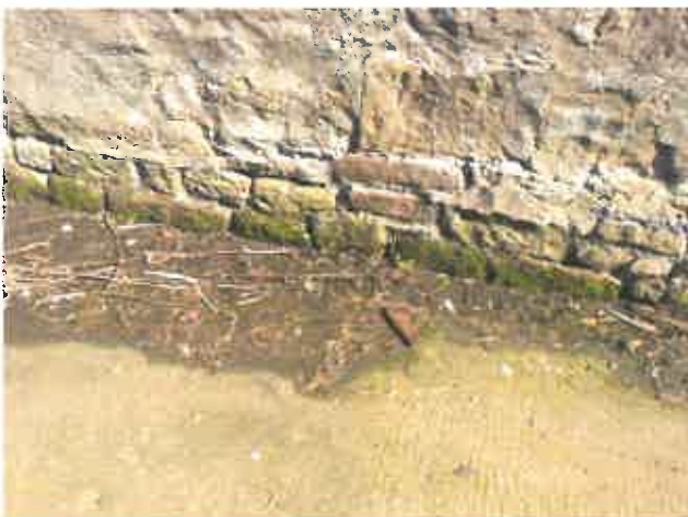
PL33 (Left) showing mortar degradation to base of wall. PL34 (Right) showing hole damage and hairline cracking to west elevation.
