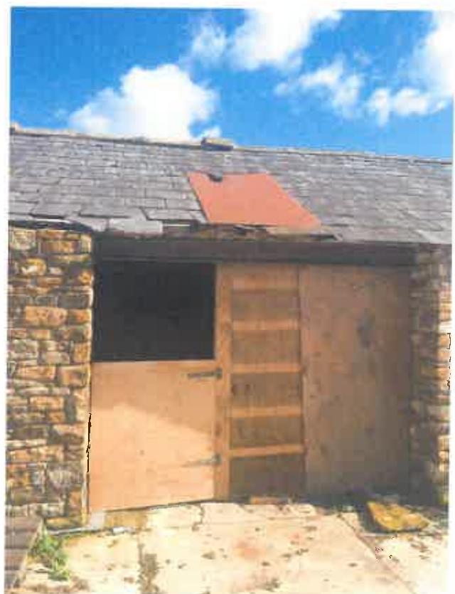
PL44 (Left) showing empty structural opening. PL45 (Right) showing ad – hoc gate / door arrangement.
