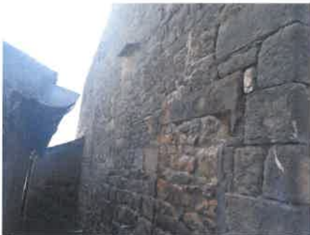
PL25 (Left) showing condition of the east elevation gable wall with degraded mortar and patch repairs. PL26 (Right) showing cracking to east elevation gable wall.
