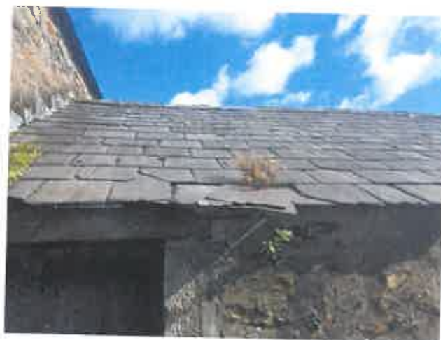
PL2 (Left) and PL3 (Right) showing cracked, chipped and dislodged slates along with vegetation growth.
