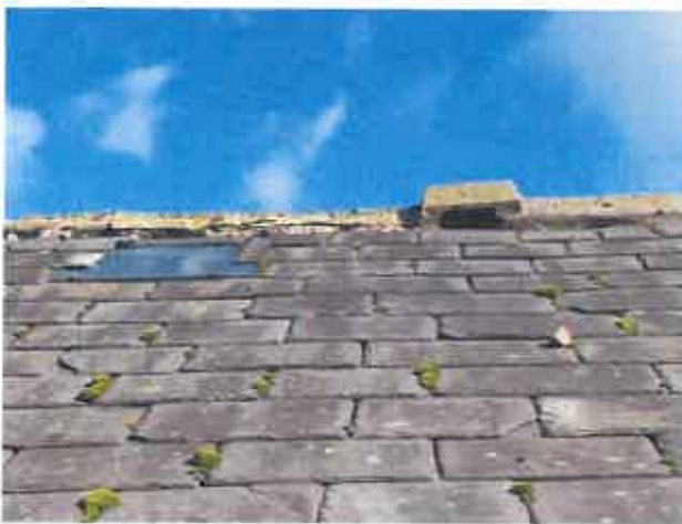
PL4 (Left) and PL5 (Right) showing degradation to ridge tiles and pointing as well as cracked, chipped and dislodged slates with vegetation growth.
