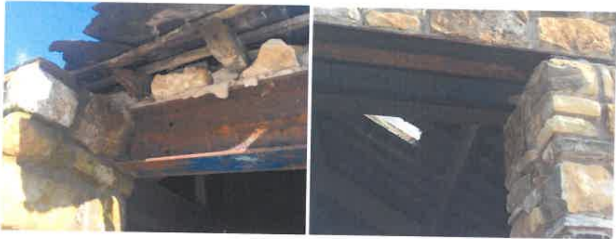
PL50 (left) and PL51 (Right) showing rust and corrosion to steel lintels above openings.
