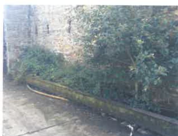
PL19 (Left) showing rust staining to below metal fixtures. PL20 (Right) showing significant vegetation growth to the base of the elevation.
