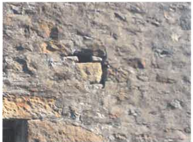
PL33 (Left) showing mortar degradation to base of wall. PL34 (Right) showing hole damage and hairline cracking to west elevation.
