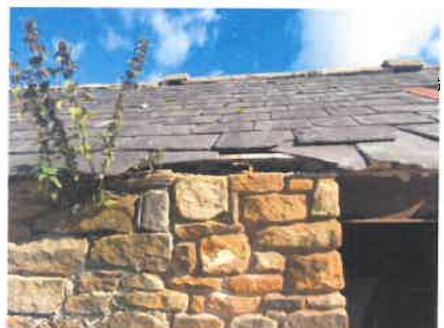
PL4 (Left) and PL5 (Right) showing degradation to ridge tiles and pointing as well as cracked, chipped and dislodged slates with vegetation growth.
