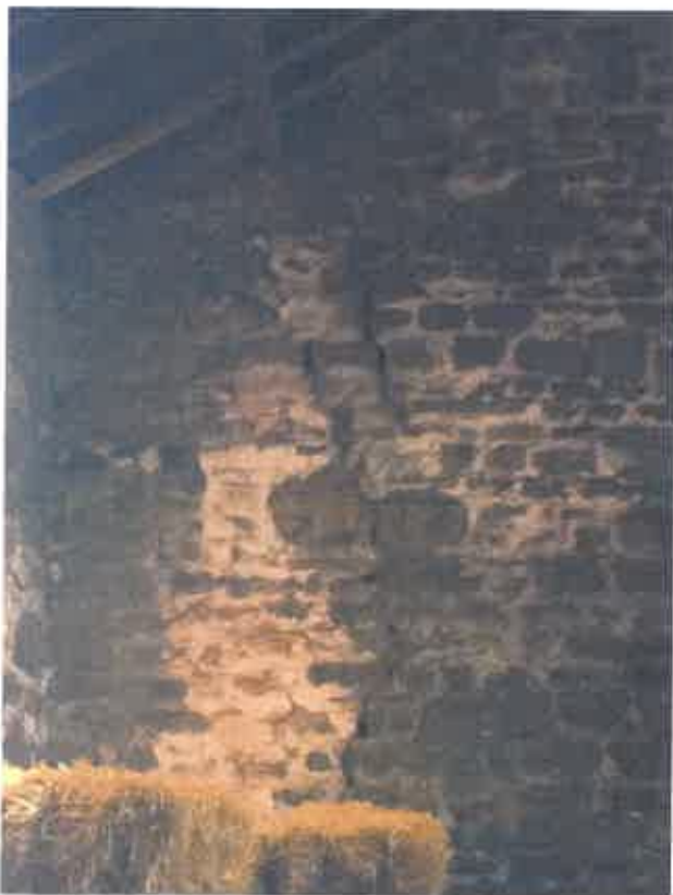
PL40 (Left) shows wall cracking to the internal face of the east gable wall within the north section of the barn and is in the same location as the external wall cracking. Minor isolated crack stitching / lateral restraint ties potentially required at this point. PL41 (Right) shows soiling and staining to internal walls.
