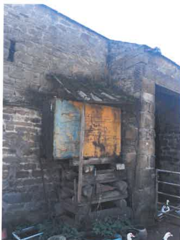
PL17 (Left) showing area of cracking to eastern side of north elevation. PL18 (Right) showing dilapidated ad-hoc structure, used to store water tank, which is to be demolished.
