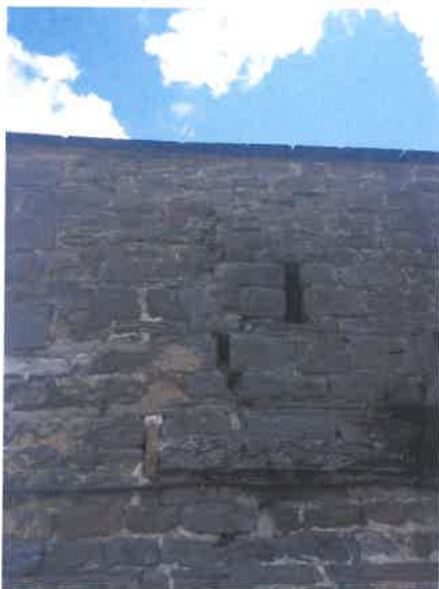
PL17 (Left) showing area of cracking to eastern side of north elevation. PL18 (Right) showing dilapidated ad-hoc structure, used to store water tank, which is to be demolished.
