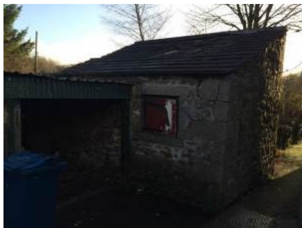
PL26 (right) showing the existing coal bunker and
