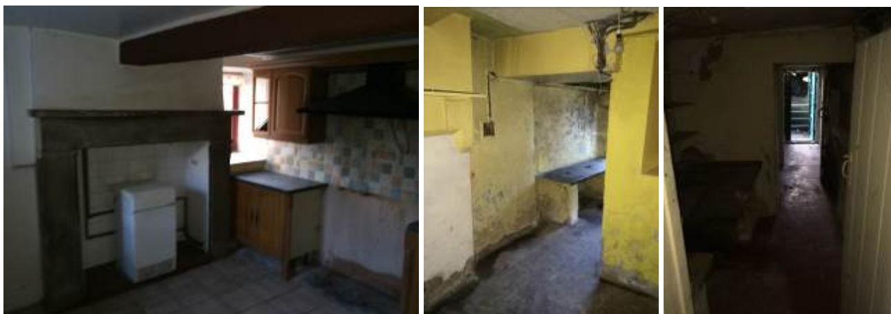
PL10 (left) image from within the existing kitchen. PL11 (middle) and PL12 (Left) taken within the existing utility room and pantry areas.
