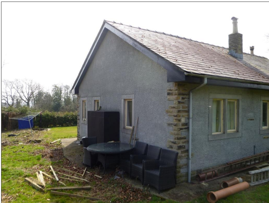
Plate 9: East end gable with well sealed windows and no access potential around the soffit
