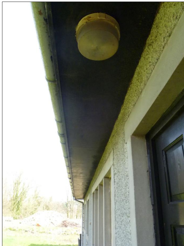
Plate 7: Underside of the soffits running along the rear side of the property were well sealed so stopping any bat access potential
