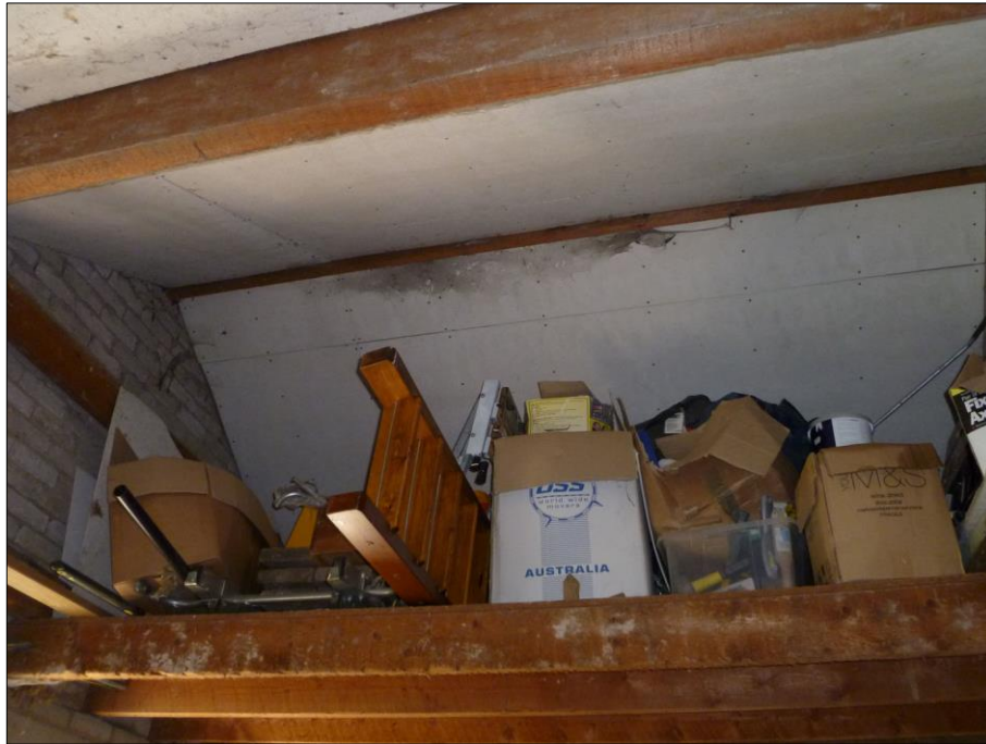
Plate 13: Internal loft space of the garage showing plasterboard
