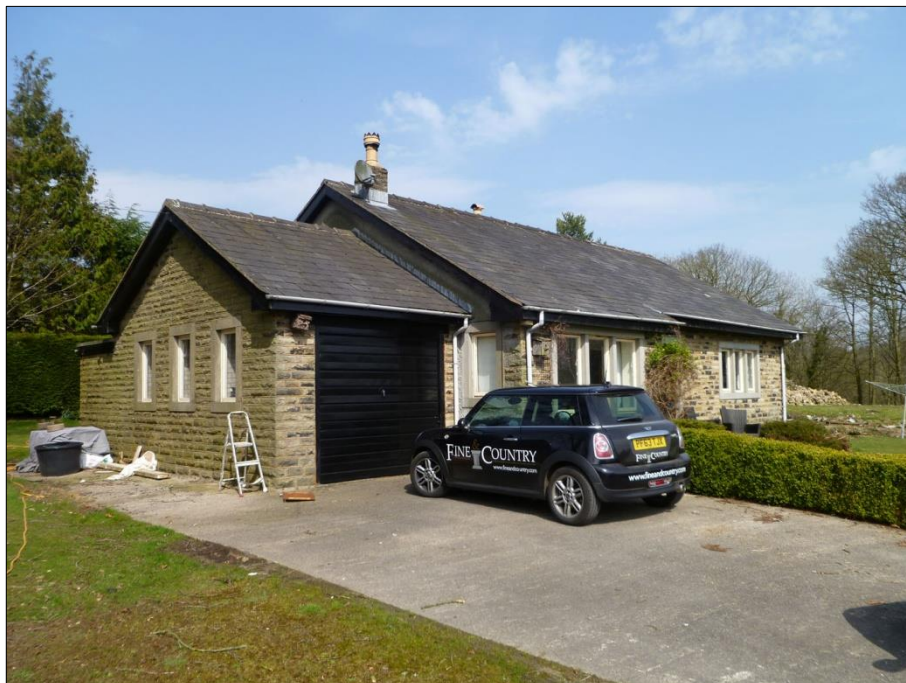
Plate 1: Front overview of the building
