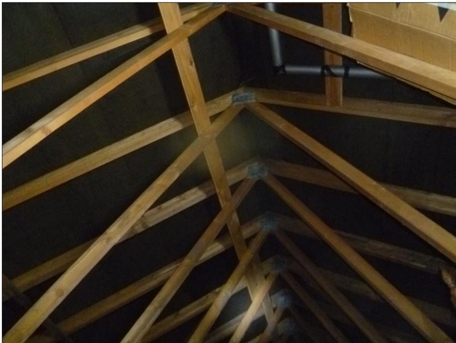
Plate 12: The underside of the roof revealed bitumen felt in good order
