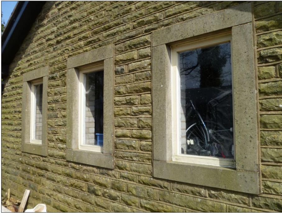
Plate 2: All the windows and doors were well sealed with no bat access potential
