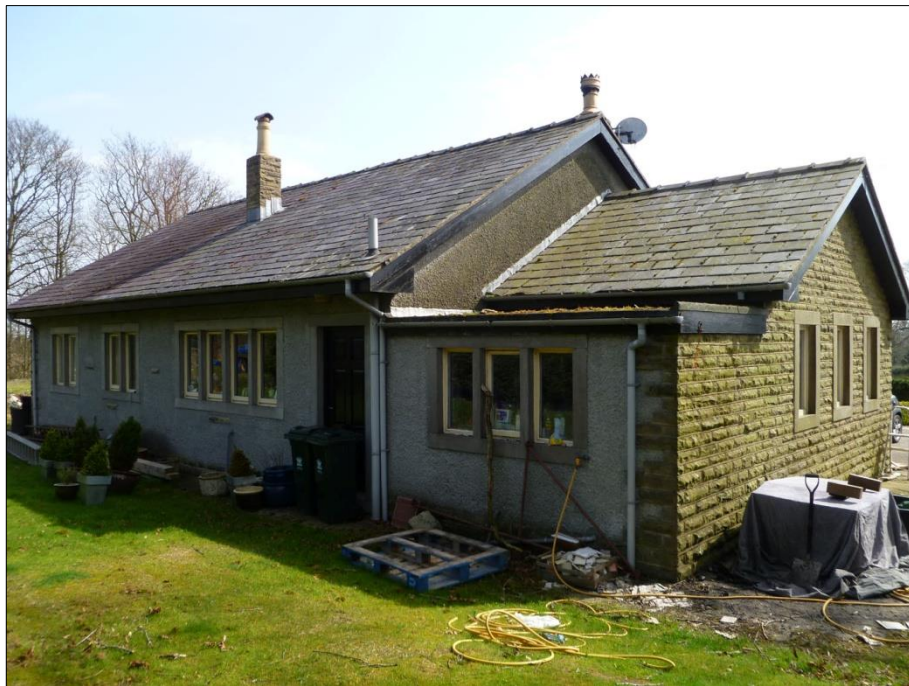
Plate 5: Rear side of the property showing a flat roof extension attached to the garage
