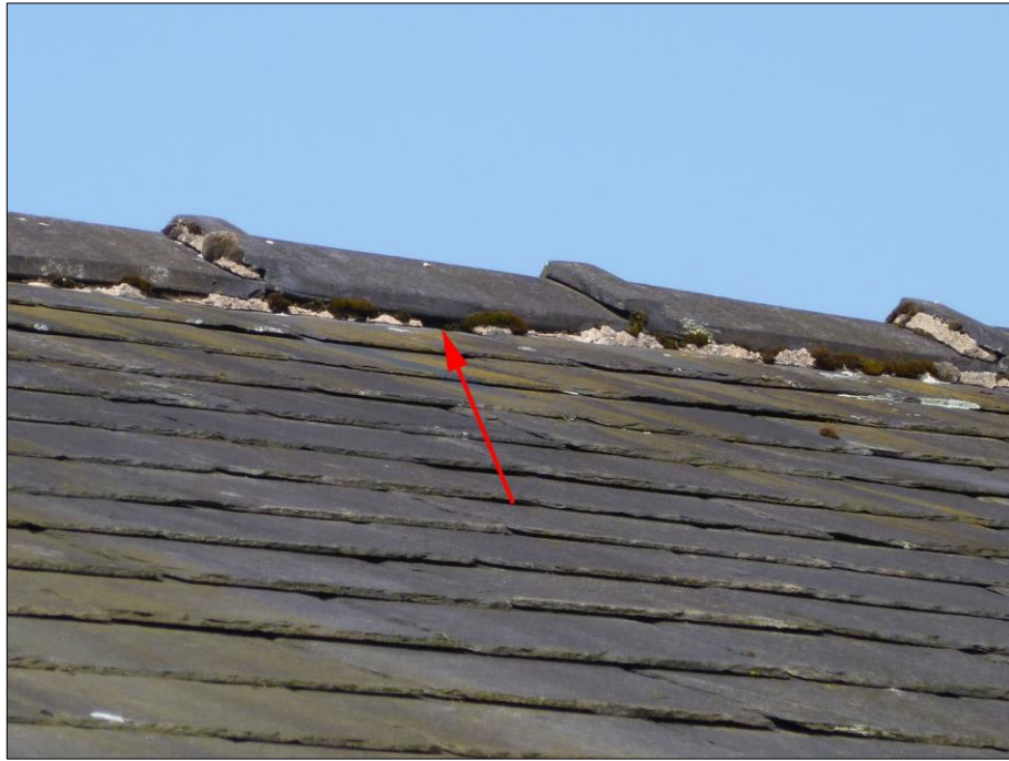
Plate 4: Potential access opportunities were observed along the ridge line of the garage section of the building
