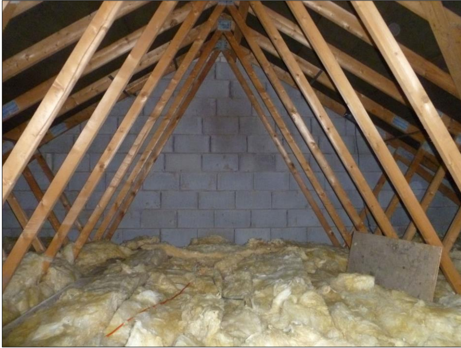
Plate 11: Internal loft space of the main building showed no bat signs or access potential
