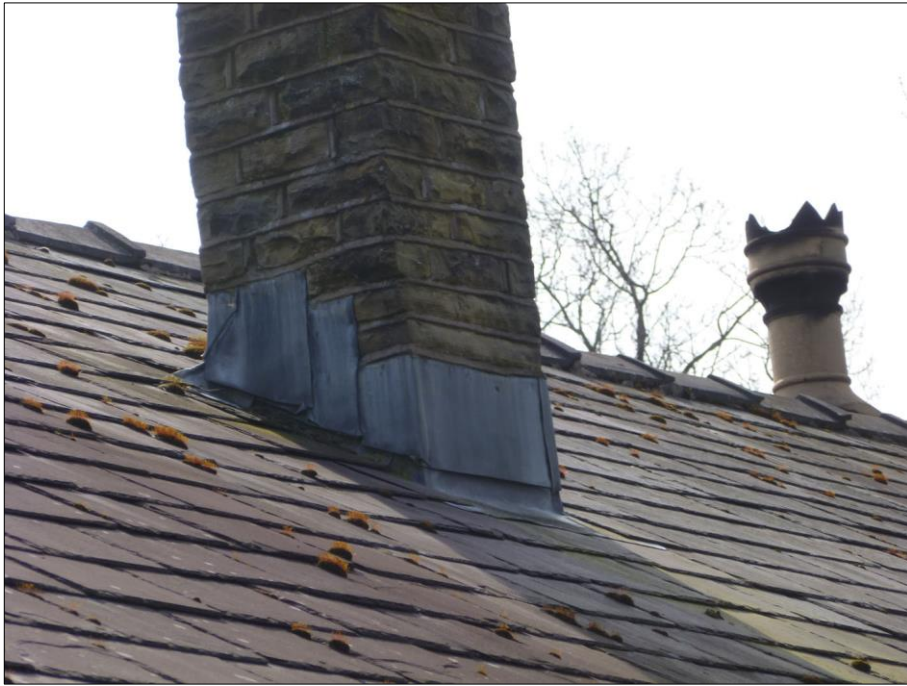
Plate 8: Rear side of the roof revealed no bat access potential
