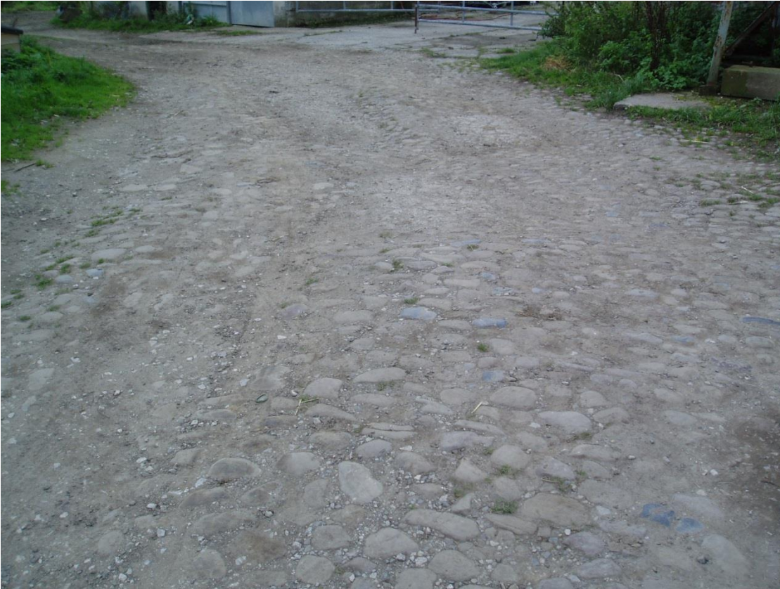
Cobbled surface of the farm yard
