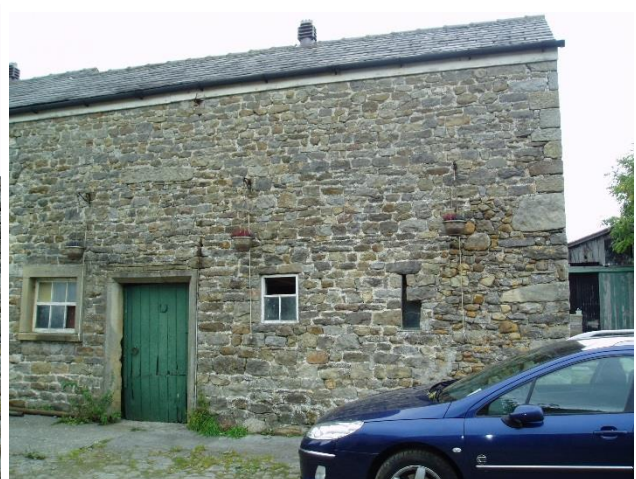
South elevation north barn
