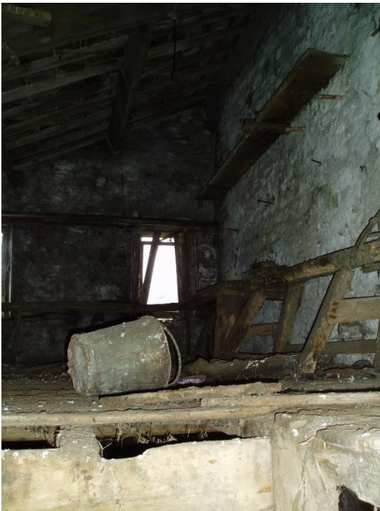
Harness room and workshop
