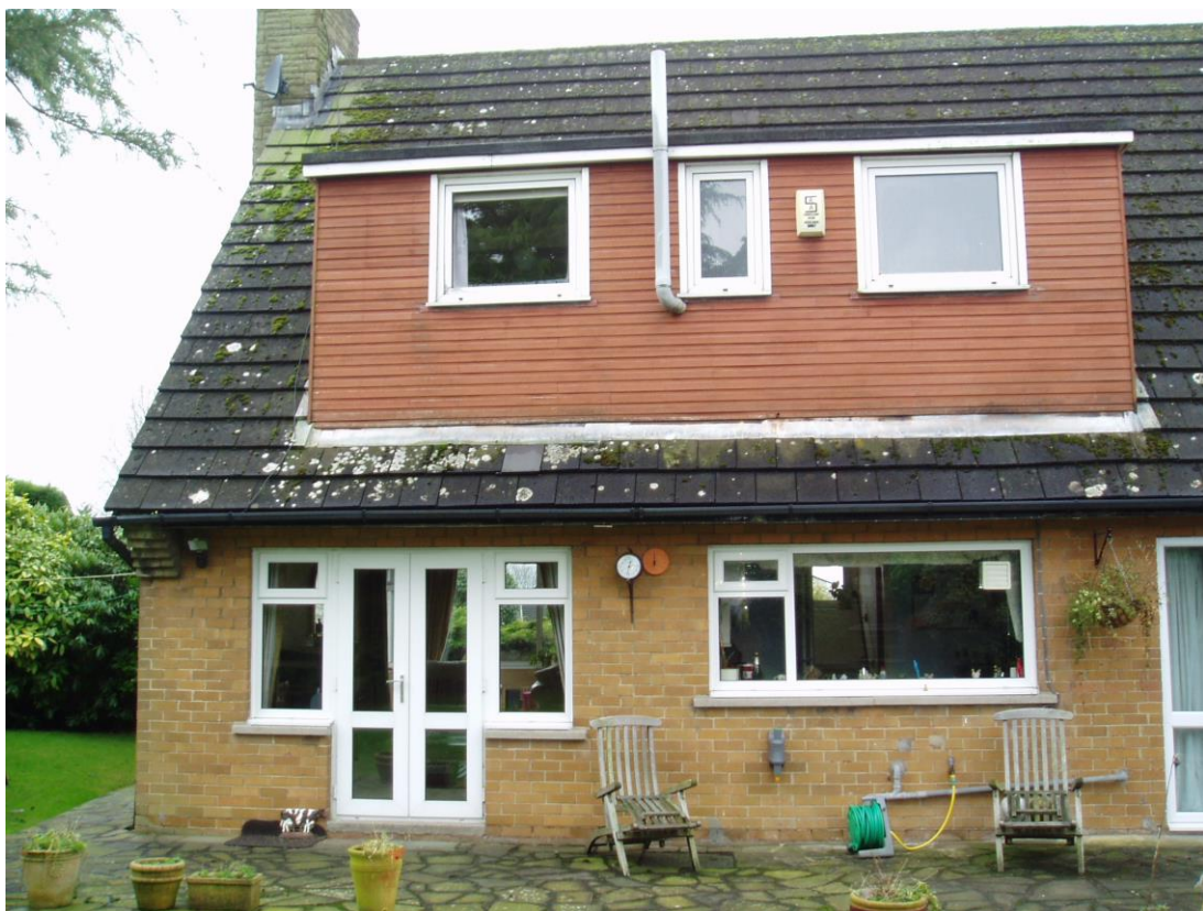
1 Existing rear dormer.
