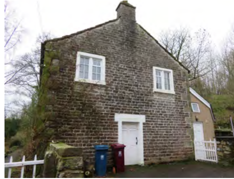
NE Elevation: Gable of Meeting room
