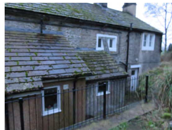
Rear of adjoining cottage beyond Meeting Room extension.
