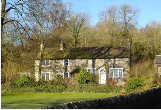
S.E Approach along access lane from Grindleton Road.
