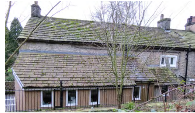
NW Elevation : Rear extension to Meeting Room & lower porch to Cottage
