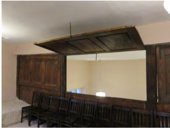
Gallery with opening timber hatches.
