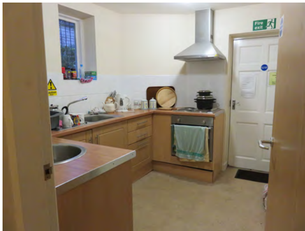
Meeting Room Kitchen in rear extension which is proposed to be taken out to provide an entrance Hall way and cloaks store.
