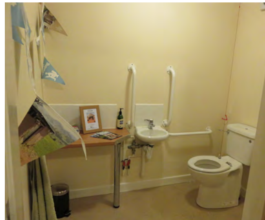
Meeting Room Disabled Toilet which is proposed to be taken out to provide access into the rear porch of the Cottage.
