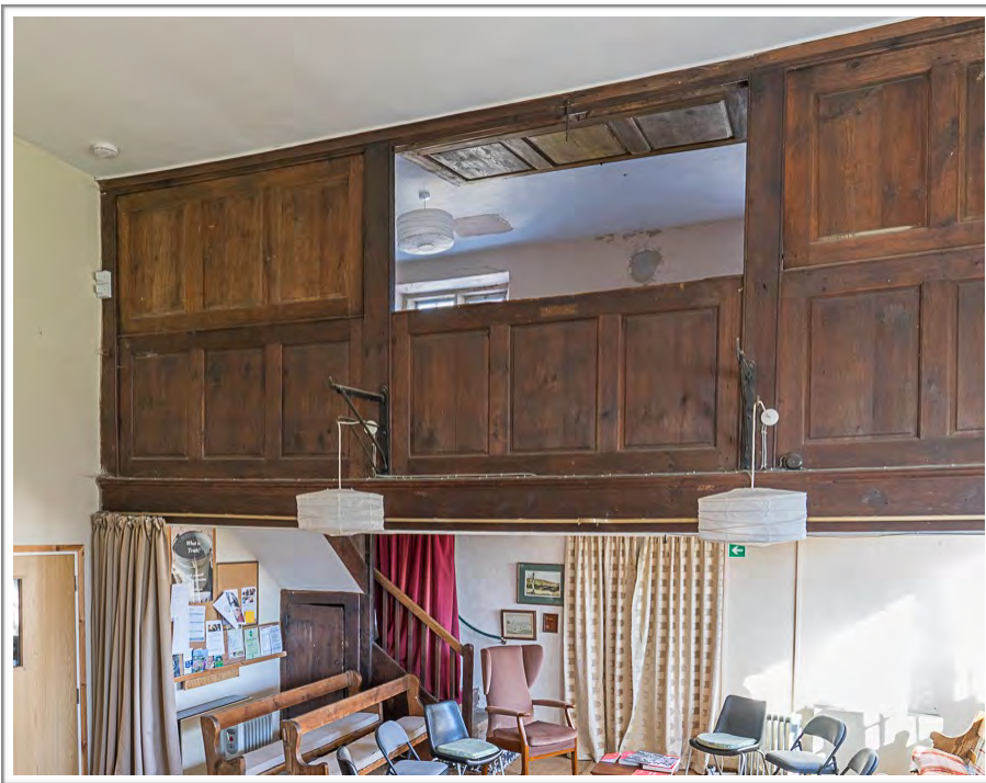
RAISED PANEL ON THE GALLERY IN THE MEETING ROOM
