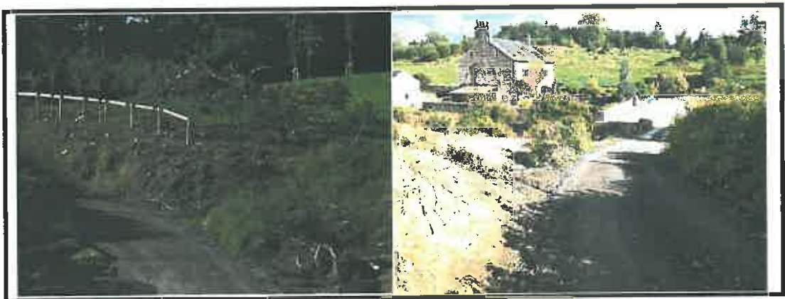
View to exist area and across bridge from car park to training centre.
