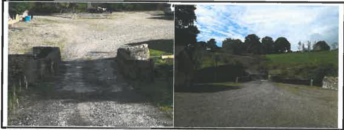
Into site and from site at bridge entrance
