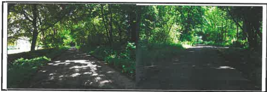
Bay 5 is approx 50m east of bay 4 at a field gate to the south side with two way flows.
