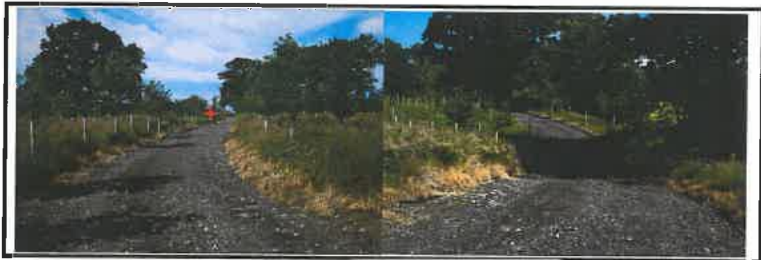
View to SW and NE as the track turns towards the road from passing area.
