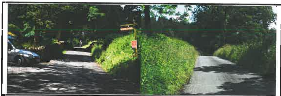
Bay 4 is a double passing bay using the farm access and field gate view west and east
