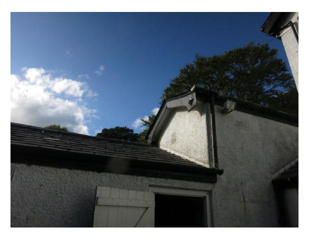
The roof has no missing or lifted slates, pointing around ridge tiles is in good condition with no gaps. Soffits and bargeboards are in good condition and close fitting.
