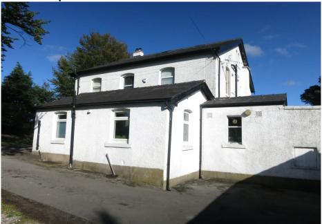
The building is a single storey extension to the main house with a slate double pitched roof. A single storey block built garage with double pitched slate roof is also included within development plans.
