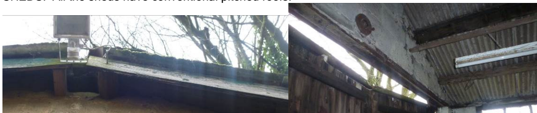
Shed 1- Corrugated fibre sheet over timber purlins
