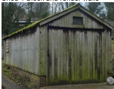
Shed 4 timber and brick plinth
