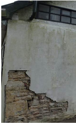
Workshop gable wall showing stone render and Painted brick.
