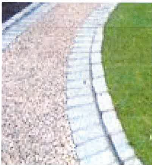
Limestone chippings with stone sett edging.
