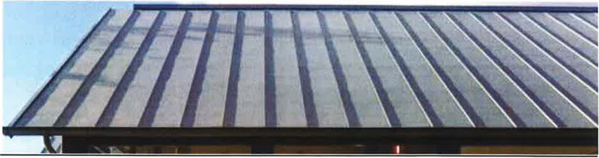
Standing seam grey metal roof.
