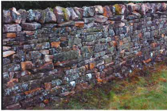
1.5m high stone wall.
