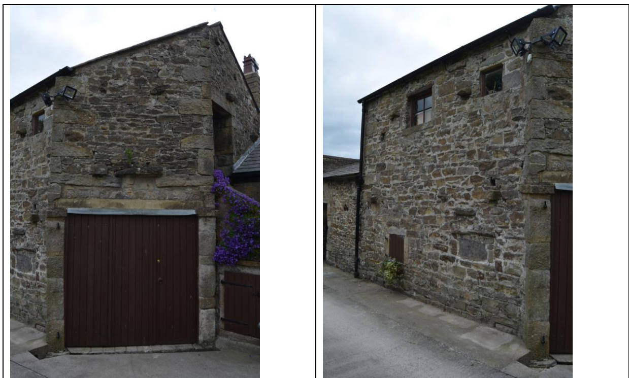
"Trap House" showing door to be retained and windows and walled up window to be opened up at Ground Floor Level
