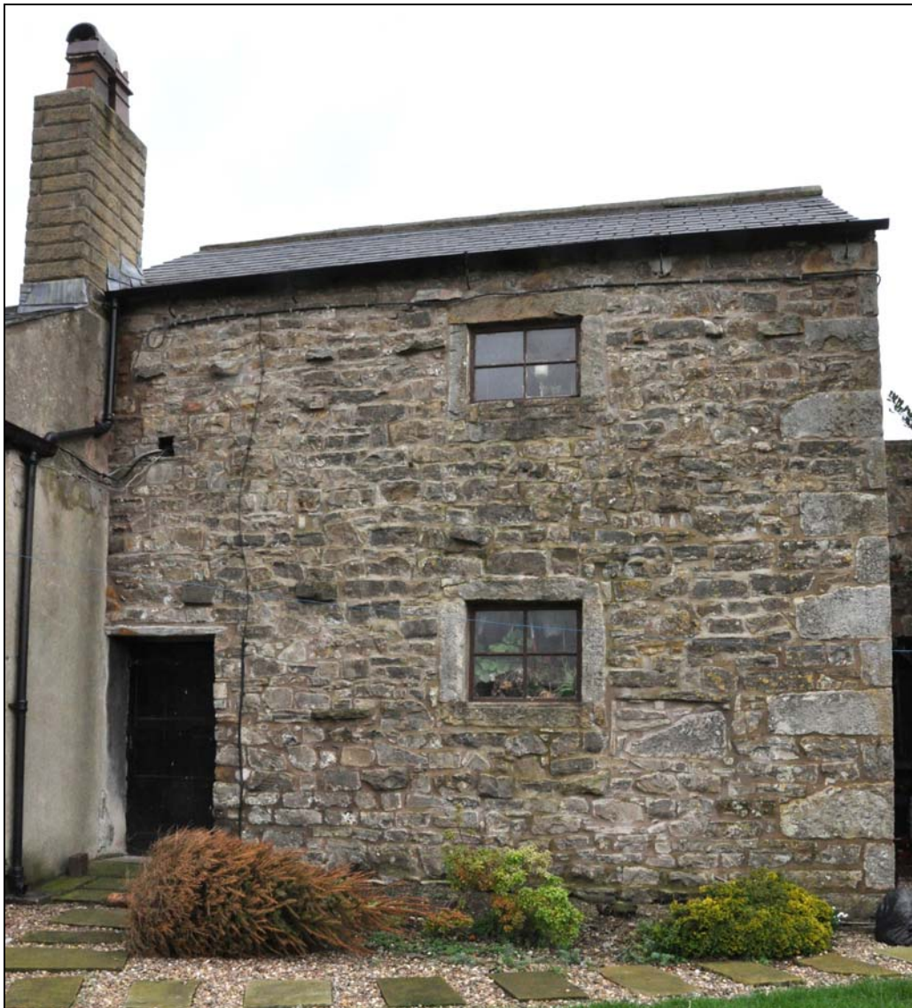
Photo 8: Front elevation of trap house with inserted doorway
