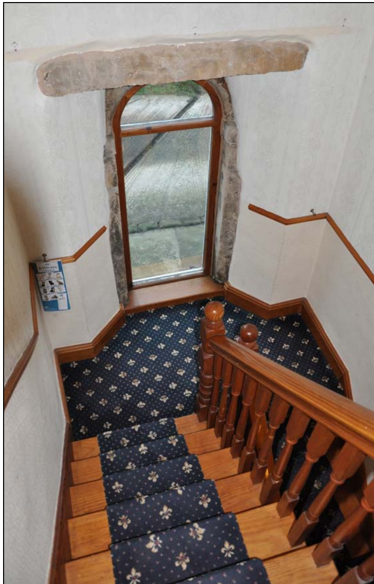
Photo 7: Modern staircase and original rear window opening (frame replaced)
