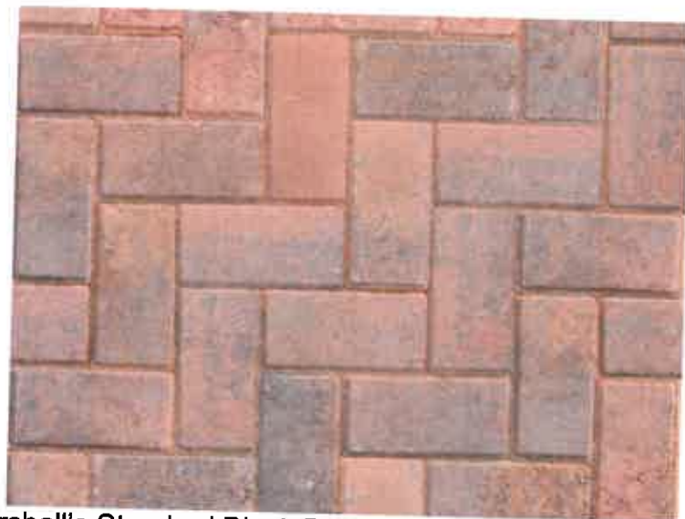
PI.3 Marshall's Standard Block Paving Brindle colour for the private car parking areas
