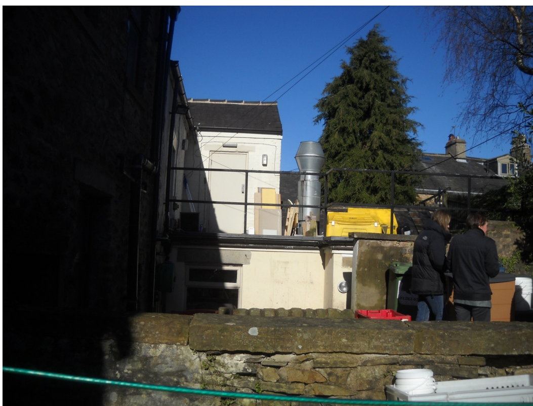
Photo. 6 View north-west from rear of No. 4 Vicarage Fold towards existing kitchen of The Freemasons Arms
