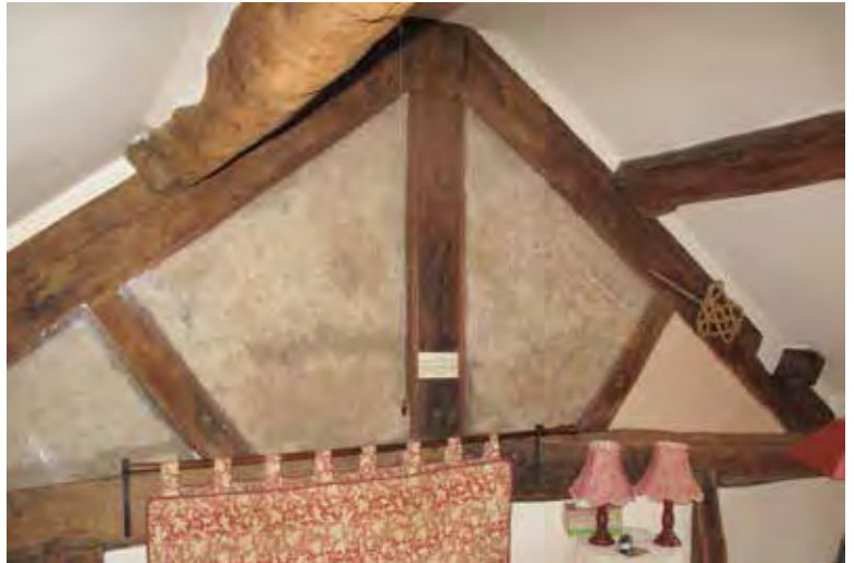
Photograph 42. The eastern roof truss, now visible in the cottage bedroom, retains wattle and daub infill.
