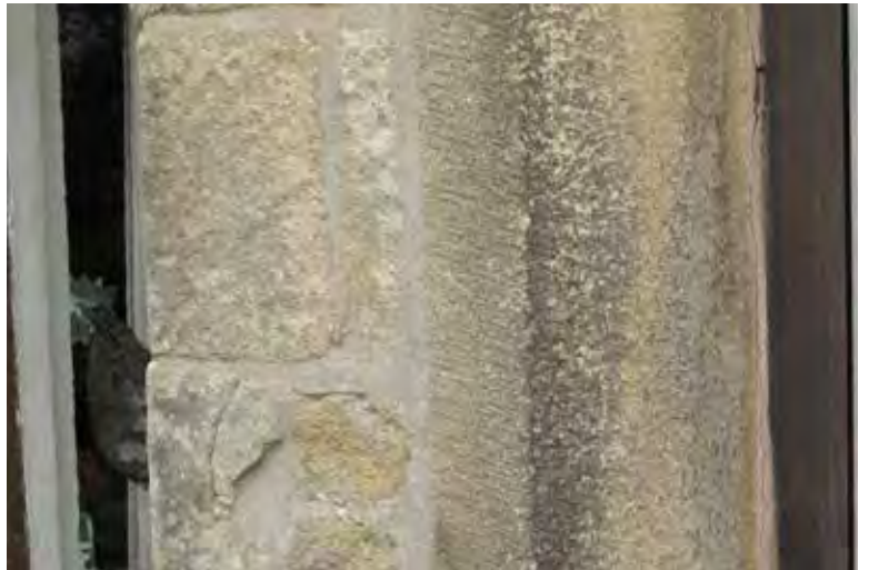
Photograph 11. Tooling on the stone surround to the front door confirms that it is a mid / late 19th century alteration.
