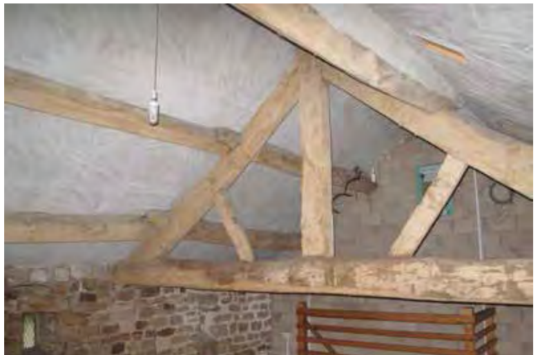
Photograph 39. The first floor of the camping barn.
