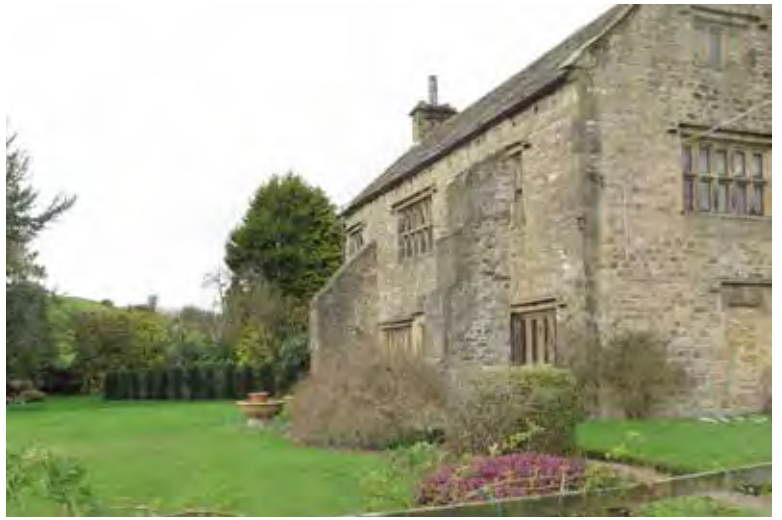
Photograph 9. The south elevation viewed from the private access track.
