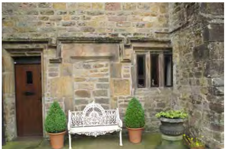
Photograph 16. The blocked doorway probably dates from later in the 17th century. Its hood mould is moulded and it seems to have been inserted between two existing windows.
