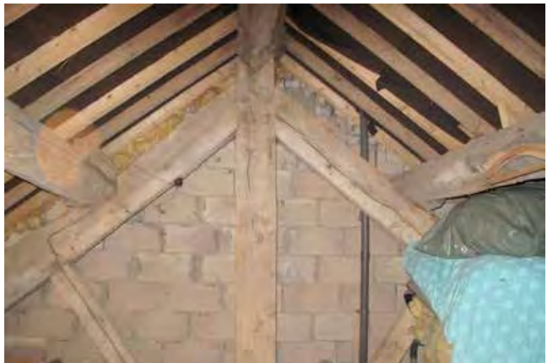
Photograph 43. The middle roof truss, visible in a first floor storage loft.
