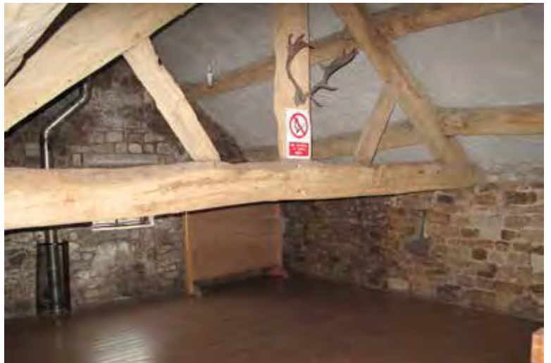
Photograph 38. The first floor of the camping barn.
