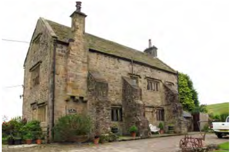
Photograph 15. The north side of the house. The corbelled chimney served a first floor fireplace that is now covered and may have been removed. There are fewer first floor windows on this side of the house and they lack transoms.
