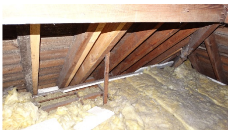
Figure 5: Main roof internal
