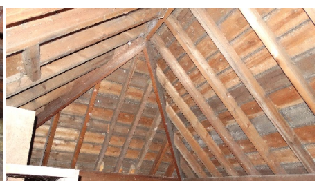
Figure 6: Main roof void
