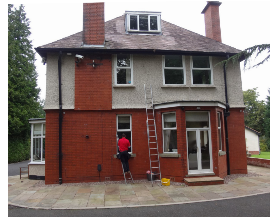
Existing elevation, approached on arrival
