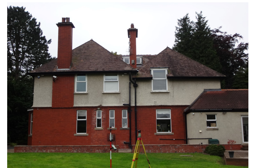
Existing elevation seen on approach
